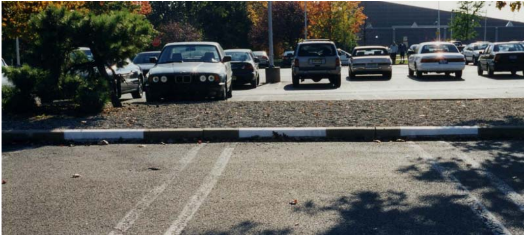
Figure 5.1(a) Coating on Concrete Curb on Busch Campus
