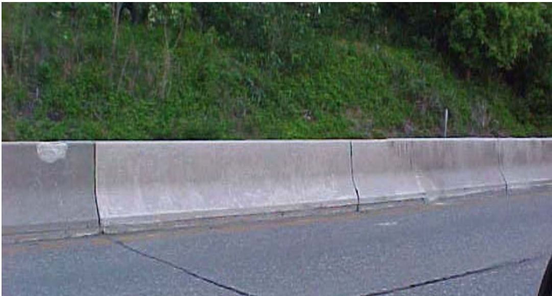
Figure 5.2 Coating on Route 1 South, Close-Up View
