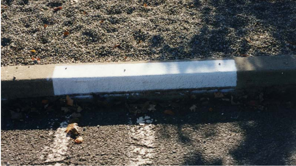
Figure 5.1(c) Coating on Concrete Curb on Busch Campus, a Close Up View
