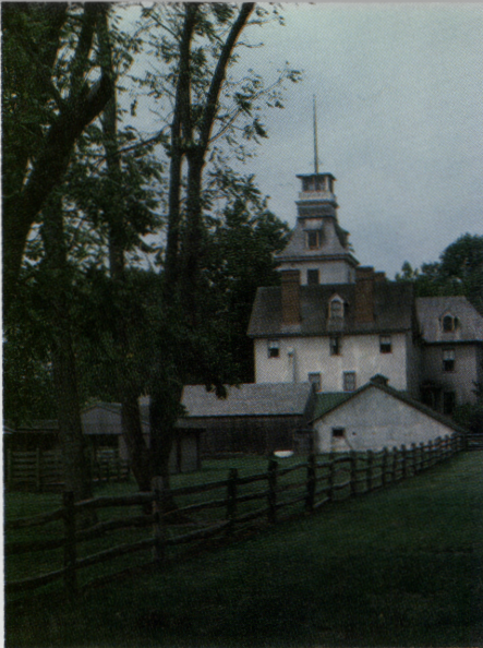
This Early-19th-century mansion located in the center of Batsto is one of the interesting buildings within the restored village.
