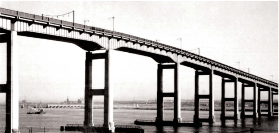
The Edison Bridge did not win any aesthetic awards, but its design was true to the doctrine of functionalism in which Morris Goodkind strongly believed. By the late 1930s, the era of adding extraneous decorative details to bridges was over. Clean lines, graceful curves, linear shadow lines, and the repetition of simple shapes such as floor beam extensions to support the sidewalks and the vertical stiffeners of plate girders, were viewed as aesthetically pleasing representatives of the "pure form" of engineering science. The bottom chord of the girders was left flat and deepened at the supports, distinguishing it from the more expensive curved type that was winning appearance awards. Source: NJDOT.
