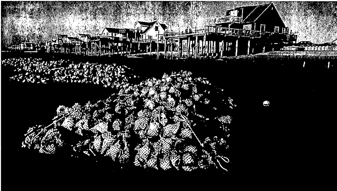
Figure 22: Intertidal shell bag reef pictured shortly after construction in at Reed's Beach. April 2014.
