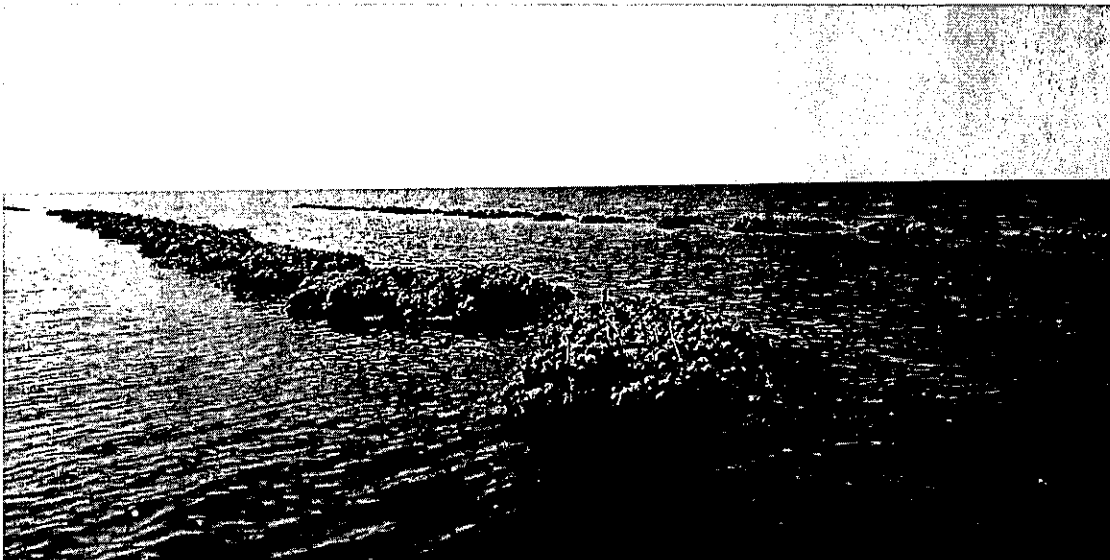
Figure 25: Cooks Beach intertidal shellbag reef shortly after installation. 2019.
