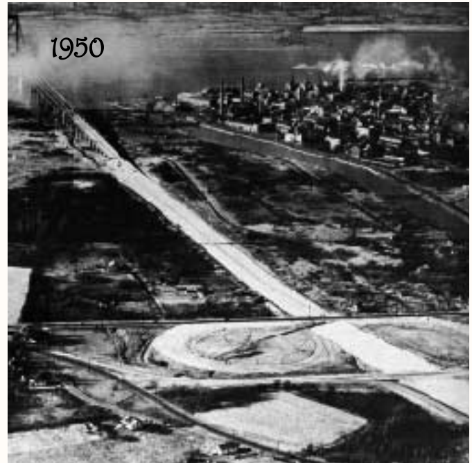
Interchange 1 and Turnpike mainline grading in Salem County (1950); Delaware Memorial Bridge in background.
