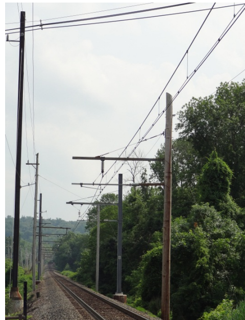
Steel Poles with Concrete Foundations
