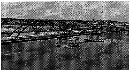
Portal Bridge: Elements of the Gateway Program, such as the replacement of Portal Bridge, have completed final design and are ready to move forward as soon as funding is secured.
