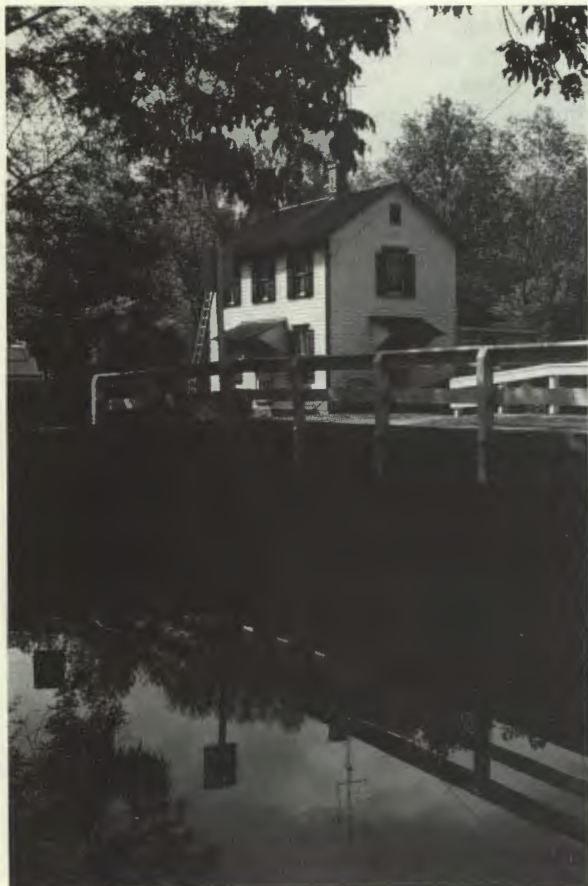
Carnegie Road Canal House in Lawrence Township.
