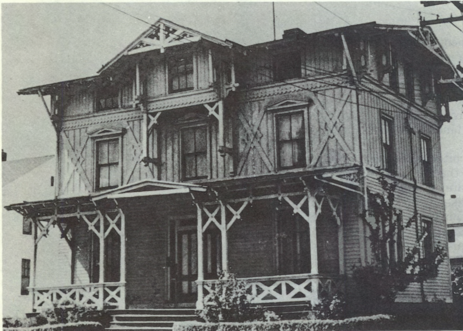
Bassett House, New Haven, Conn. 1869
