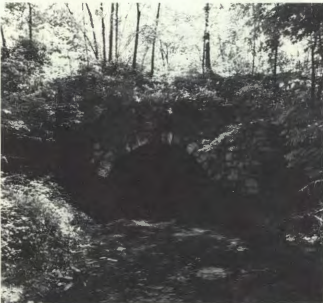
Culvert under the canal, Titusville.
