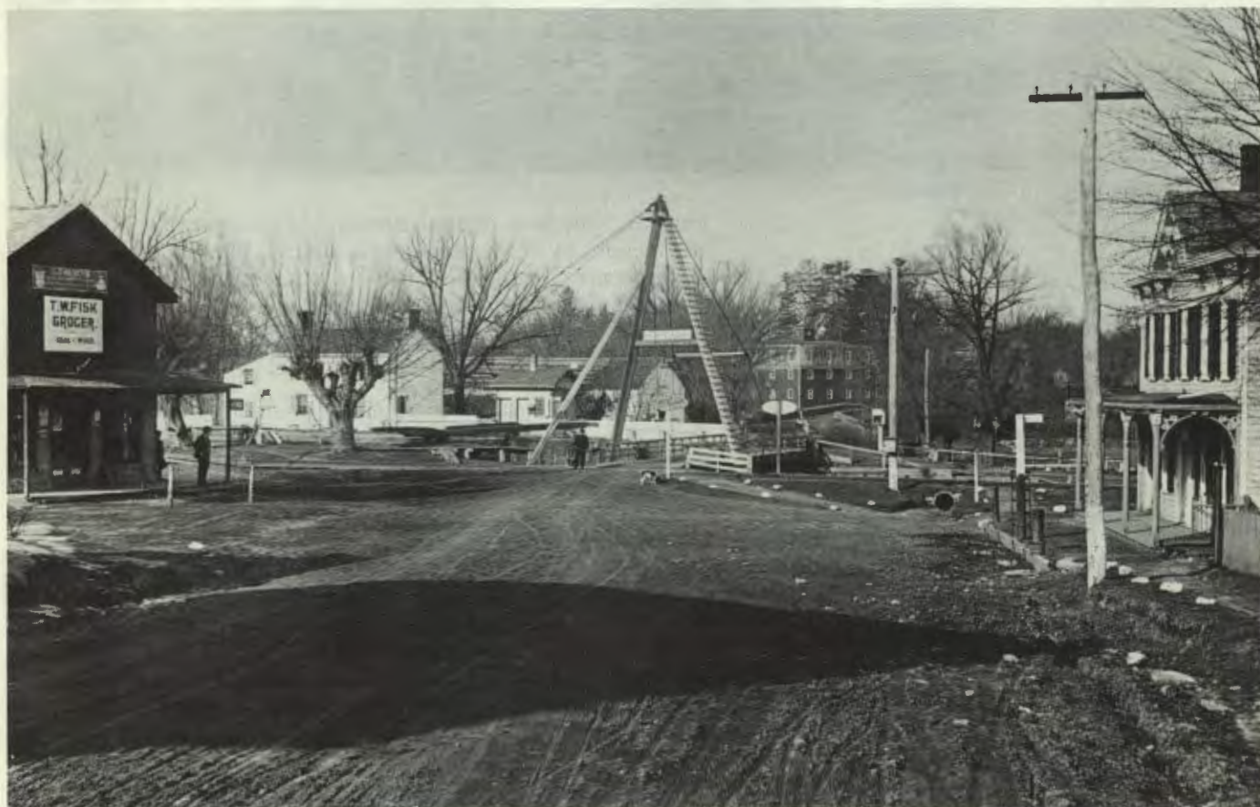
Looking south toward the canal in Kingston. The "A" frame structure was used to swing the bridge to the side when boats came. (photo courtesy of Cliff Crawford)
