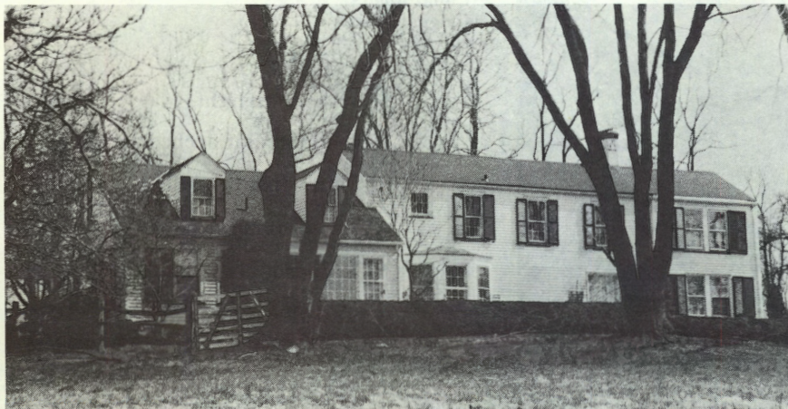
19th century vernacular house with many additions. Canal Road, Griggstown.
