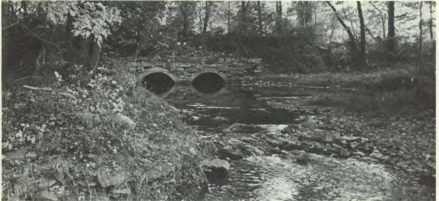
Culvert carrying Heathcote Brook under the canal.
