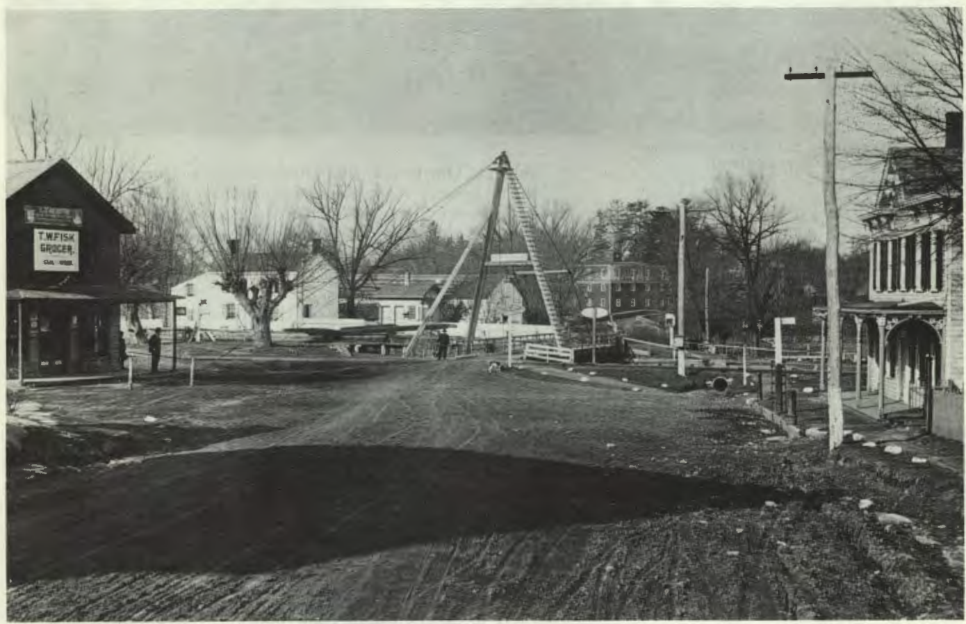
Looking south toward the canal in Kingston. The "A" frame structure was used to swing the bridge to the side when boats came. (photo courtesy of Cliff Crawford)
