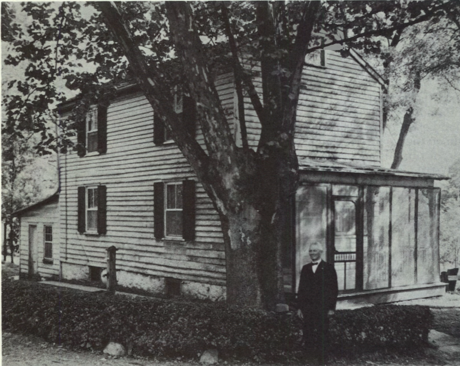
Bridgetenders House Port Mercer
