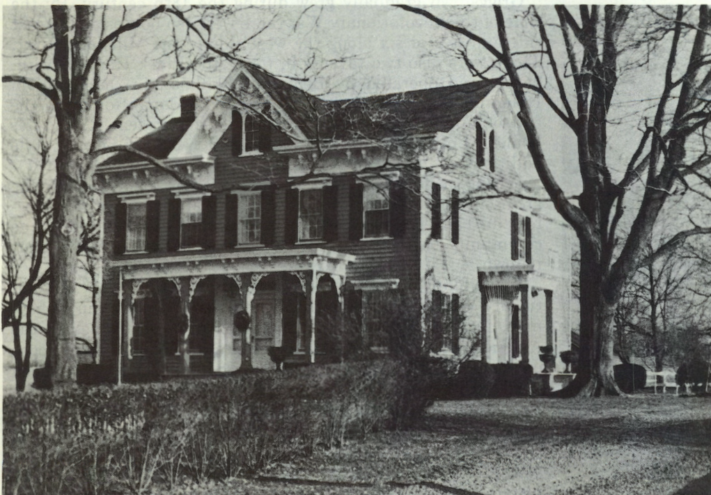
Veghte House, Canal Road, Griggstown
