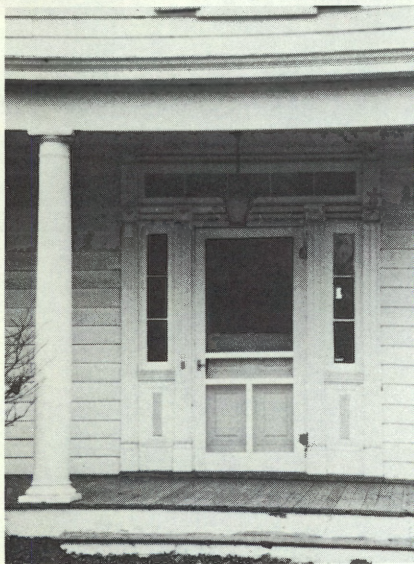
Veghte house and door detail, Griggstown
