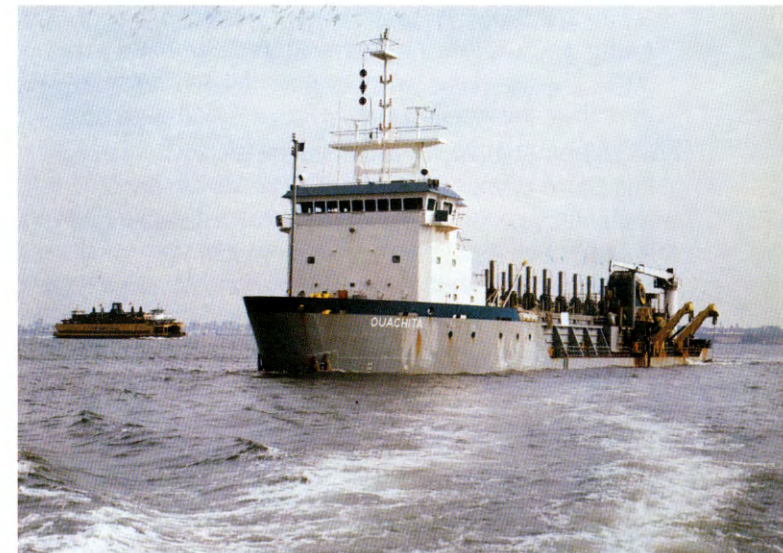
Historic dredging started in Kill Van Kull and Newark Bay in 1987. The Port Authority is paying $50 million (35 percent) of cost.
