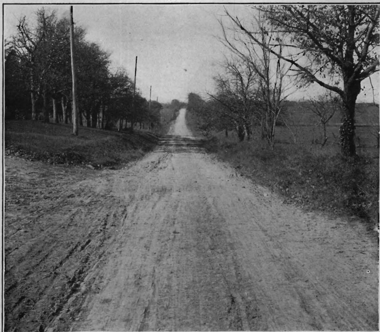
Passaic Valley road, Morris Co., before improvement.
