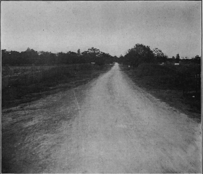
River road, Camden Co., after improvement.
