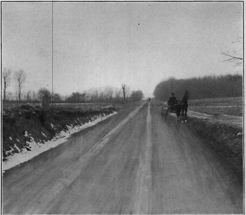
River road, Camden Co., after improvement.
