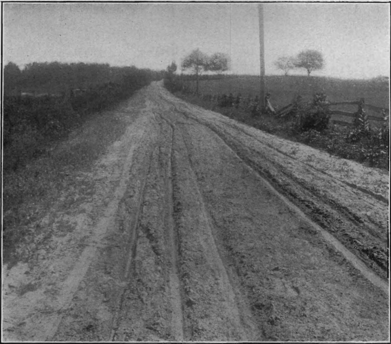
Holmdel and Marlboro road, Monmouth Co., before improvement.
