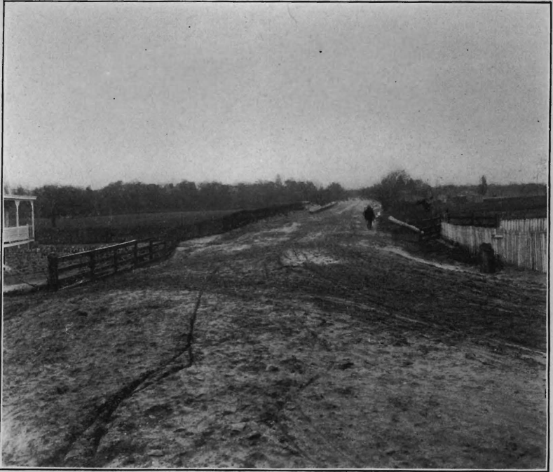
River road, Camden, Co., before improvement.
