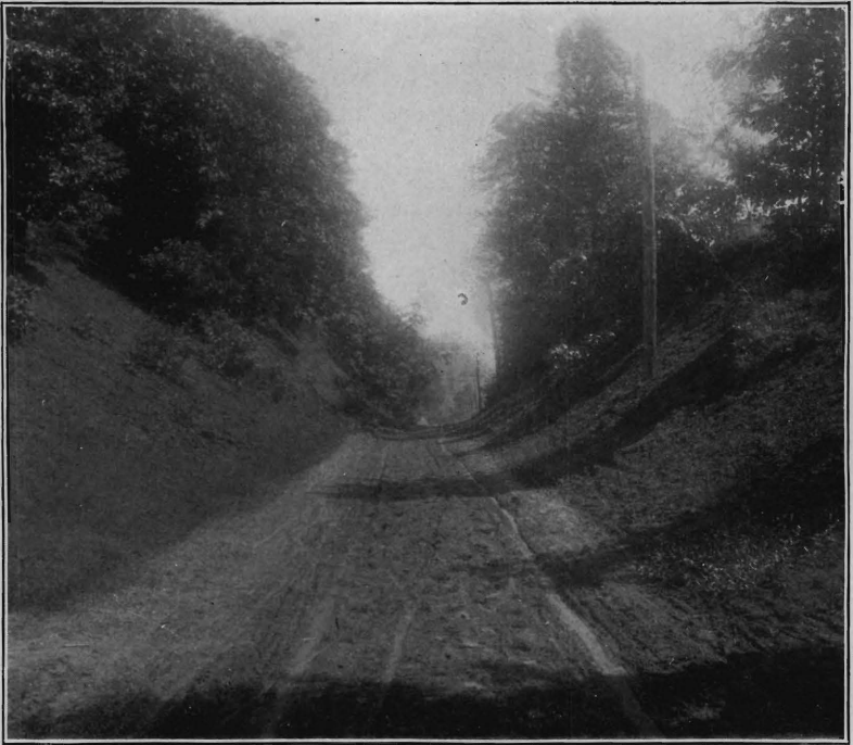
Deep cut, Holmdel and Marlboro road, Monmouth Co., before improvement.
