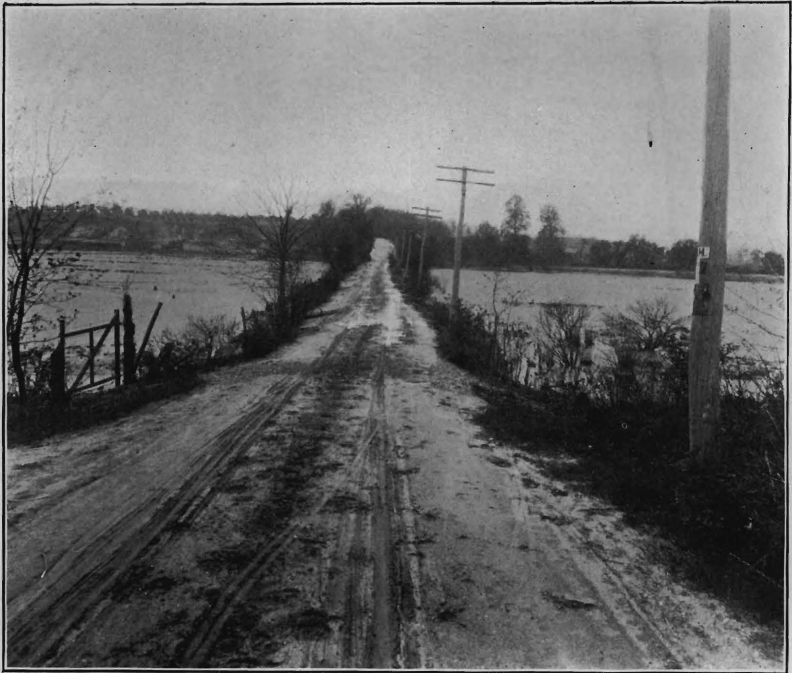
River road, Camden Co., before improvement.
