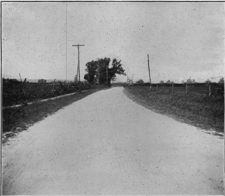
Pedricktown road, Salem Co., after improvement.
