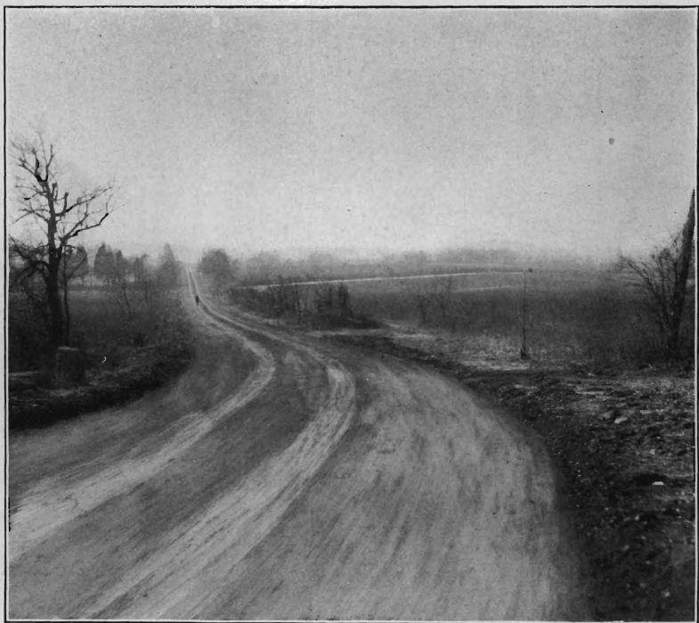
River road, Camden Co., after improvement.
