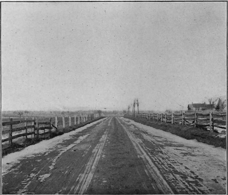
Conover's Corner and Liberty School House road, Somerset Co., after improvement.
