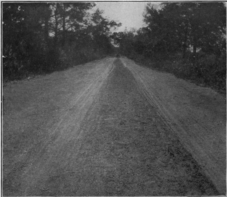
Stoy road, near Maple ave., Camden Co., after improvement.
