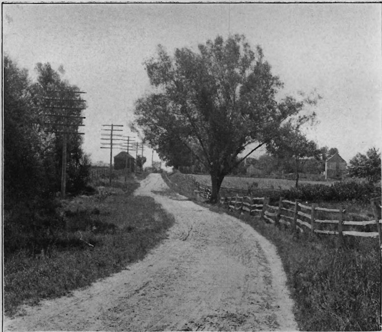
South Plainfield road, Middlesex Co., before improvement.
