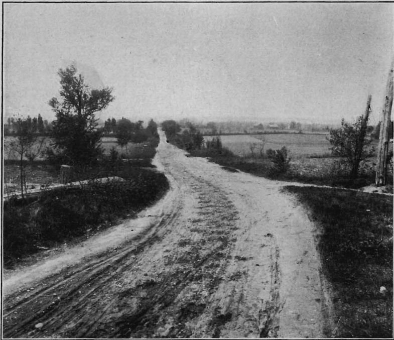
River road, Camden Co., three-quarters of a mile from county line, before improvement.
