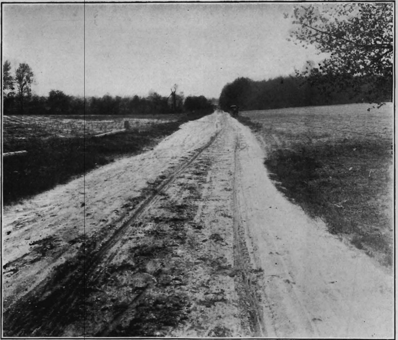
River road, Camden Co., before improvement.
