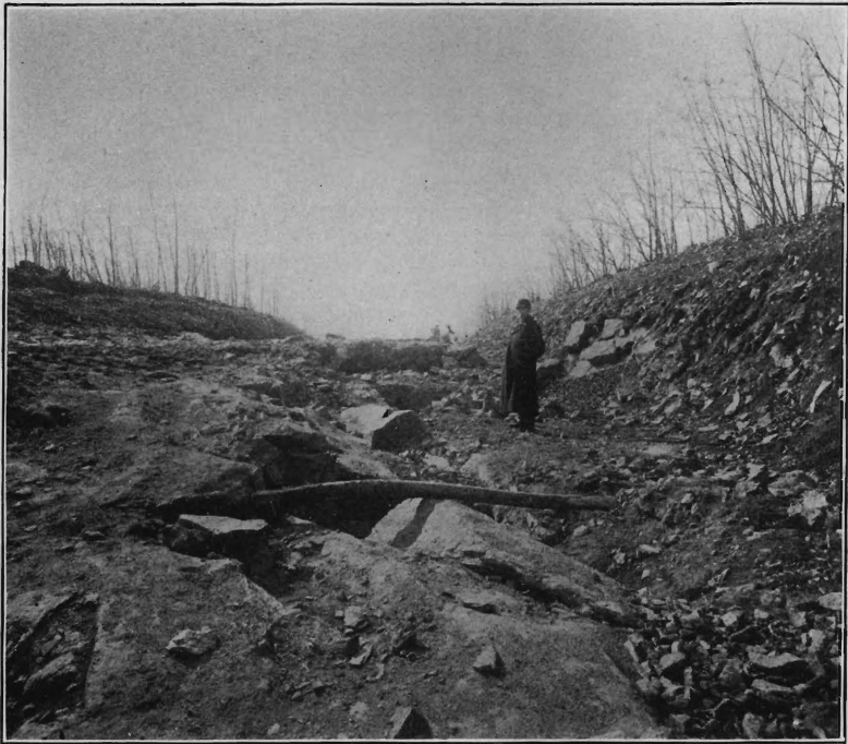
Newton turnpike, Randolph township, Morris Co., before improvement.
