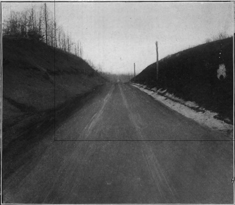
Deep cut, Holmdel and Marlboro road, Monmouth Co., after improvement.
