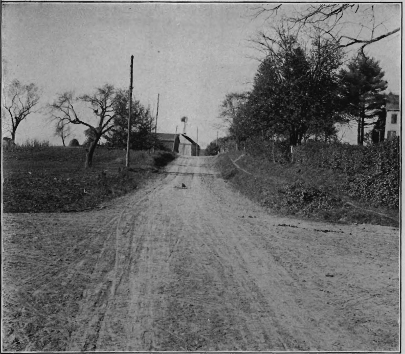
Passaic Valley road, Morris Co., before improvement
