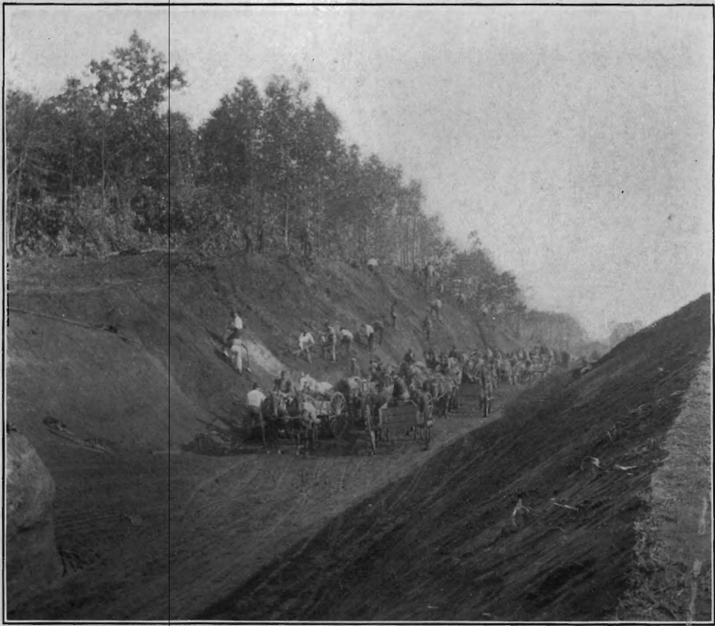
Deep cut, Holmdel and Marlboro road, Monmouth Co., during improvement.
