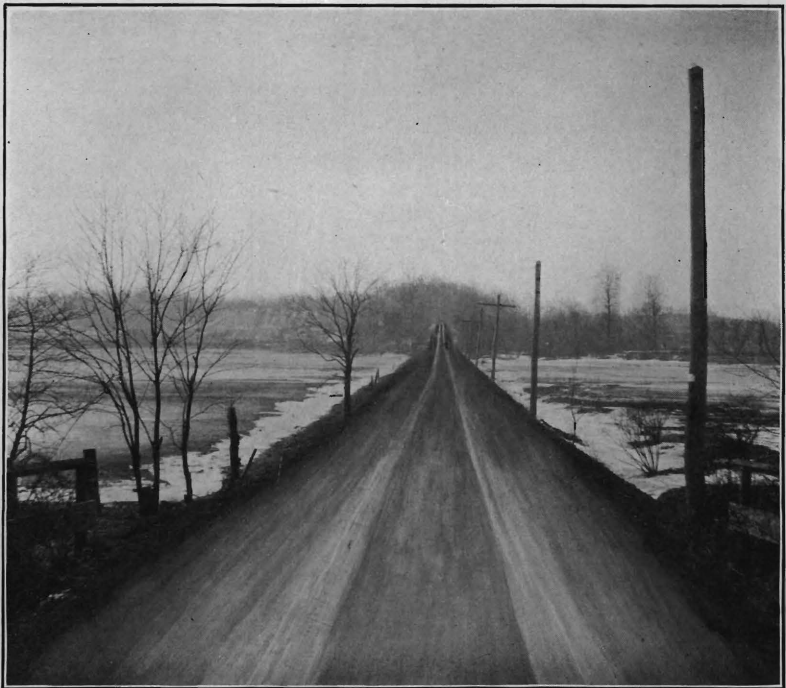
River road, Camden Co., after improvement. Cribbing on both sides.
