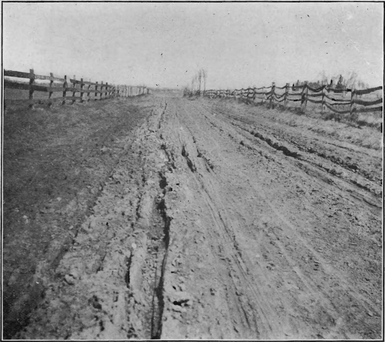
Conover's Corner and Liberty School House road, Somerset Co., before improvement.
