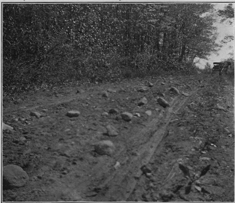
West Passaic ave., Essex Co., before improvement.
