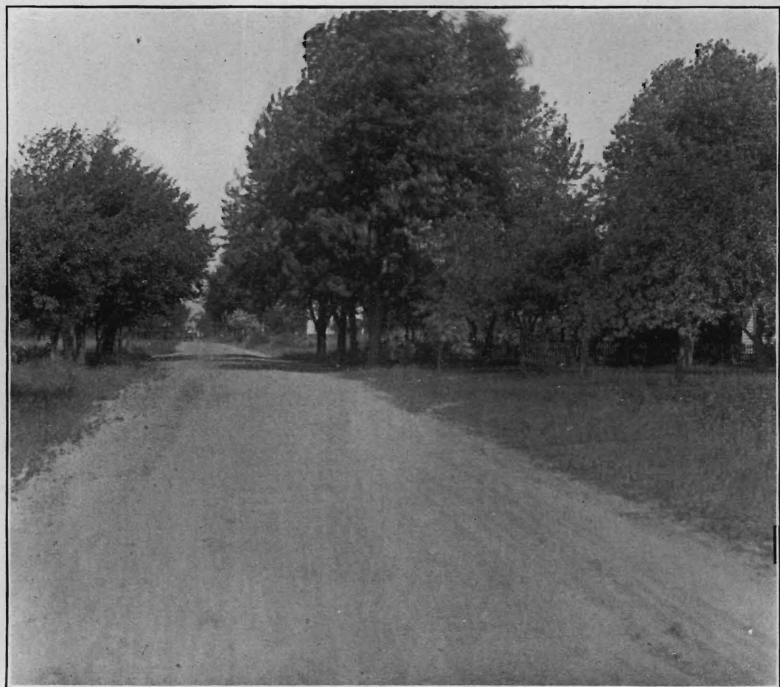
Lakewood and Point Pleasant road, Ocean Co., after improvement.
