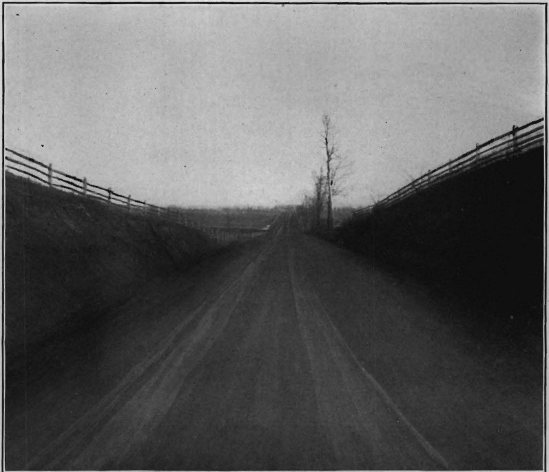
Holmdel and Marlboro road, Monmouth Co., after improvement.
