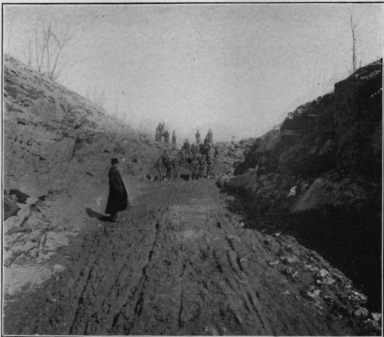
Newton turnpike, Randolph township, Till Hill, Morris Co., during improvement.
