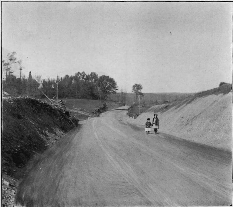
Blairstown road, Warren Co., after improvement.
