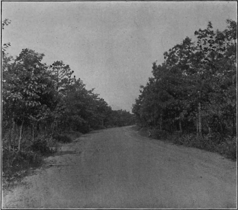
Lakewood and Point Pleasant road, Ocean Co., after improvement.
