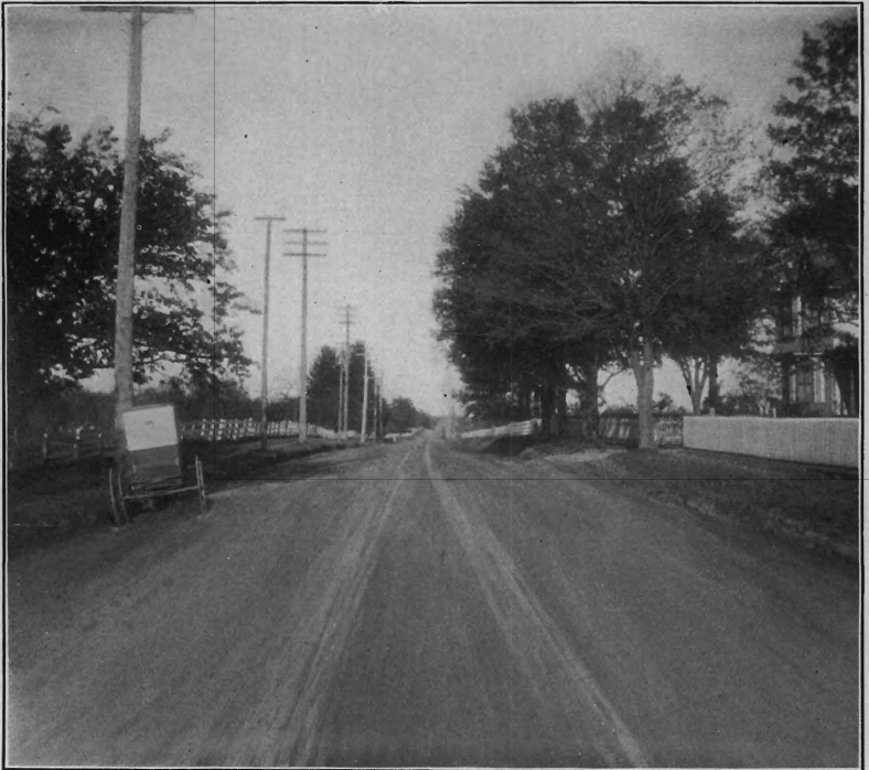
Cranbury and Pleasant Hill road, Middlesex Co., after improvement.
