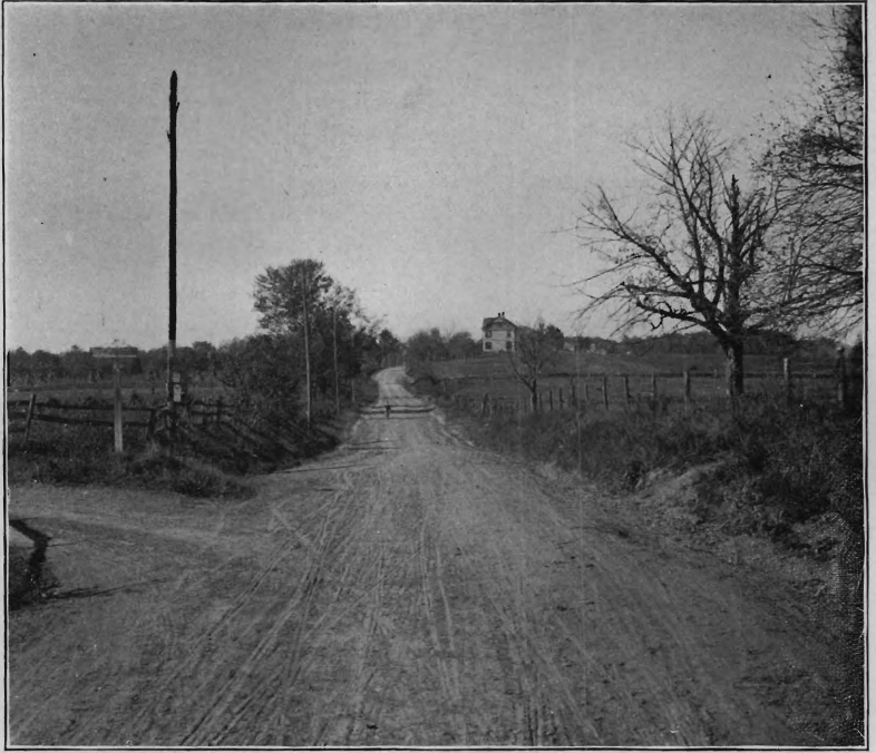
Passaic Valley road, Morris Co., before improvement.
