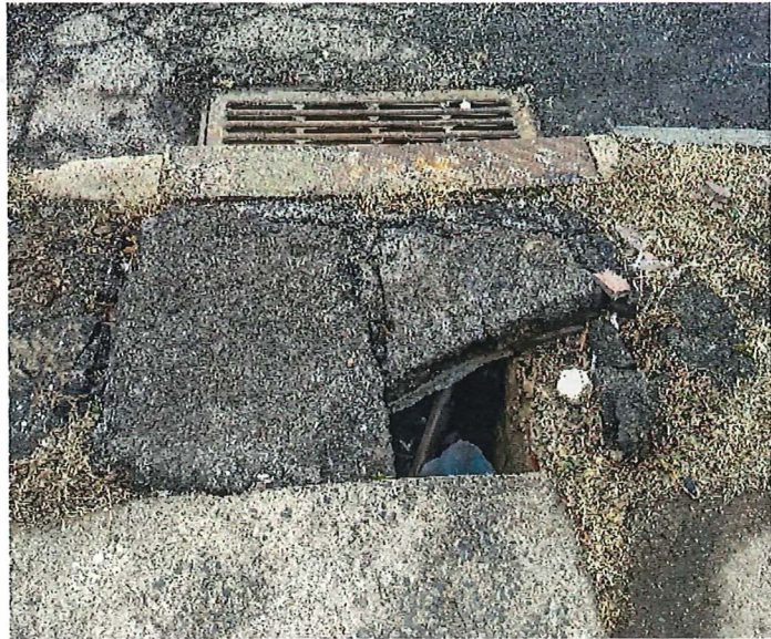
Orange City - Various Street Paving Project
