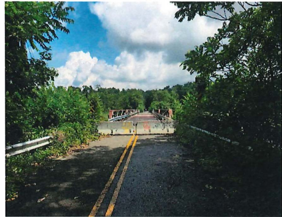
Burlington County - Centerton Road Bridge Demolition
