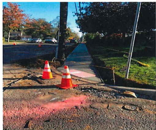
Little Silver - Branch Avenue Sidewalks
