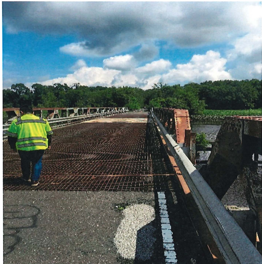
Burlington County – Centerton Road Bridge Demolition
