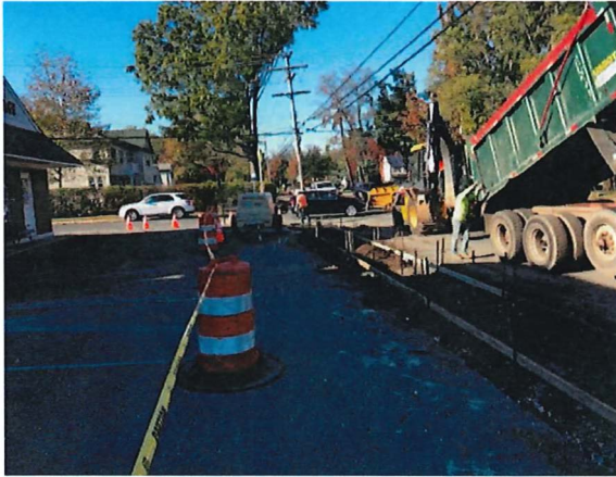
Little Silver - Branch Avenue Sidewalks
