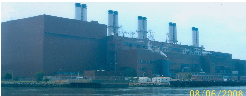
NEW YORK POWER AUTHORITY-POLETTI PROJECT
