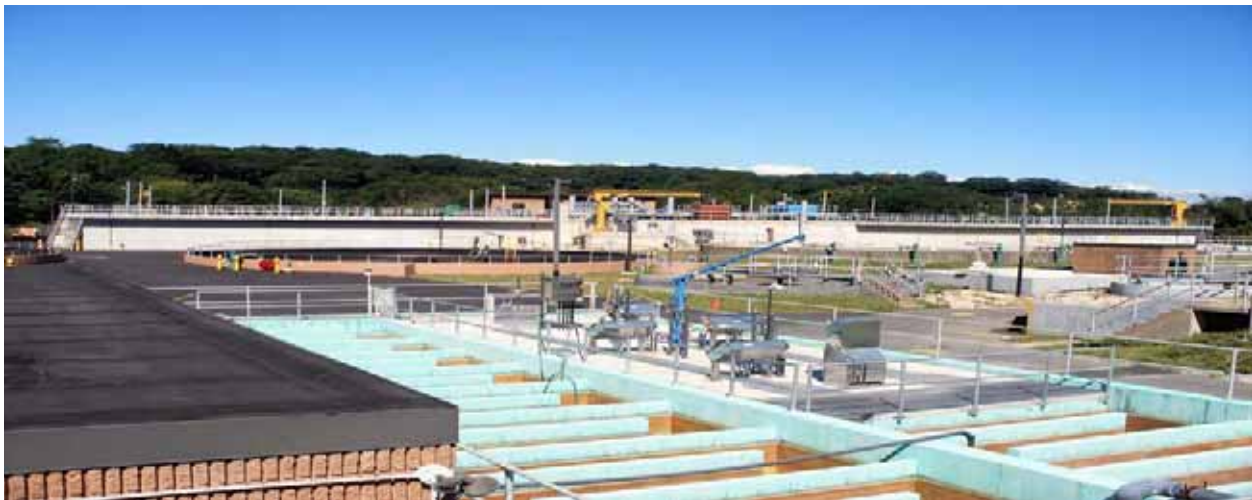
COMPLETE UPGRADED FACILITY WITH UV DISINFECTION Photo Courtesy of H2M
