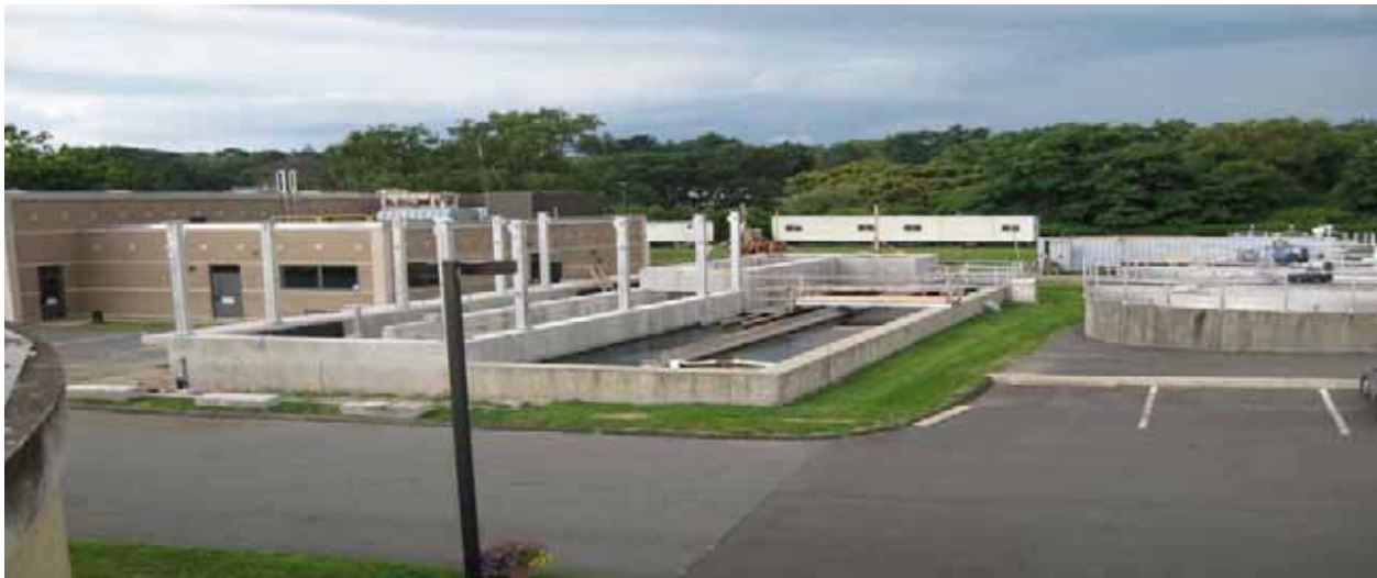
UV DISINFECTION CONTACT TANKS UNDER CONSTRUCTION
