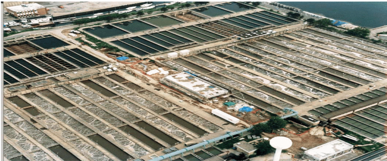
RETROFIT STEP FEED BNR Photo Courtesy of NYC DEP
