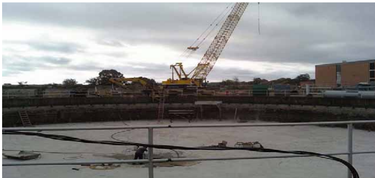
FINAL CLARIFIER UNDER CONSTRUCTION
