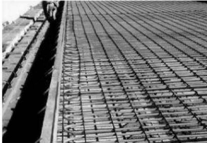
Figure 15. Amarillo, TX geothermal heating system construction: heating hoses in place ready for concrete pour
