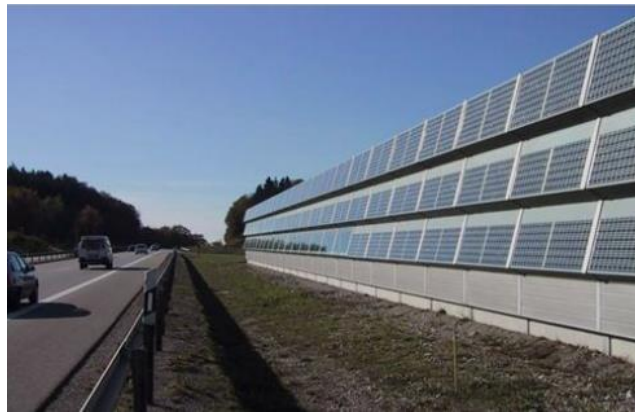
Figure 10. Photovoltaic Noise Barrier in Europe
