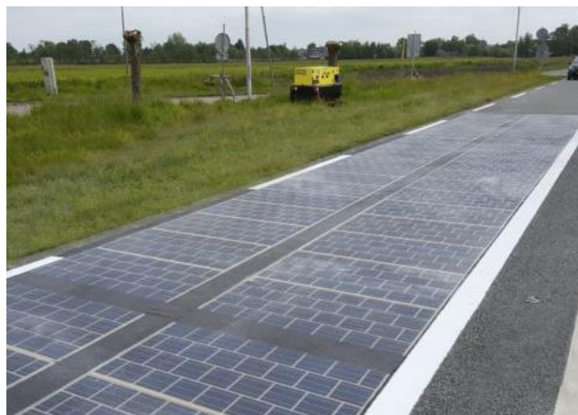
Figure 13. Solar Pavement - Wattway by Colas (France)
