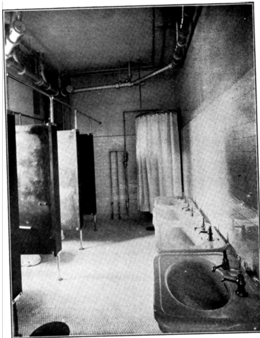
FIG. 20. Type of wash room and toilet room with shower bath in corner of new equipment.
