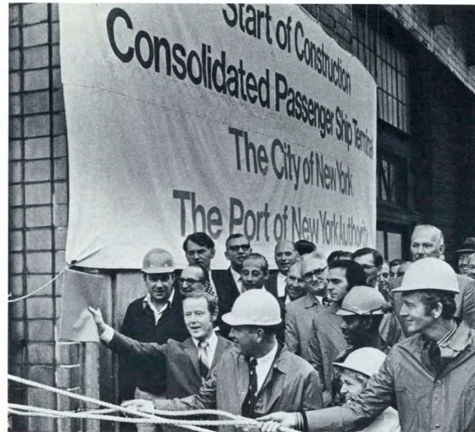
At the start-of-construction ceremony for the new Passenger Ship Terminal. Mrs. Helen Delich Bentley, Chairman of the Federal Maritime Commission, helps pull down iron railing of abandoned piers, with Port Authority Chairman James C. Kellogg, III, wearing hard hat (left), and Mayor John V. Lindsay of the City of New York (right).
