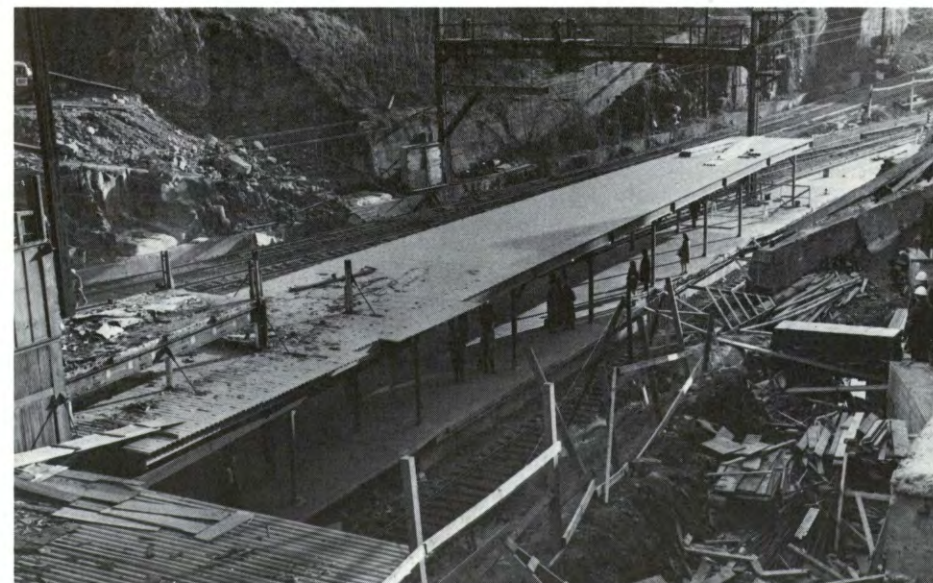
Construction proceeded on the extension of PATH platforms at Journal Square.
