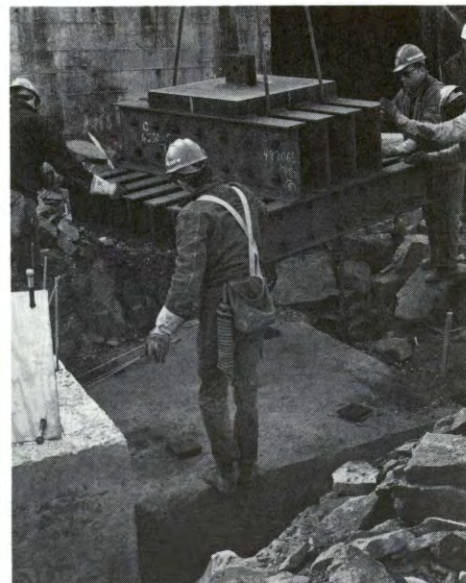
The first steel grillage is placed in the foundation.
