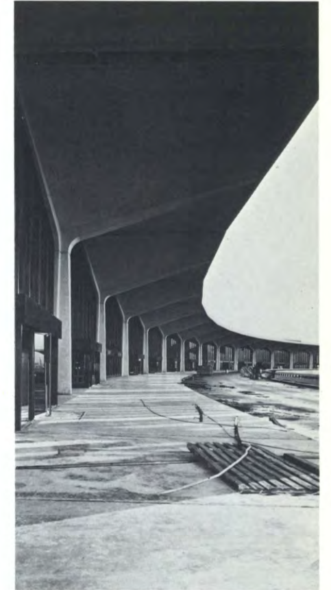
A close-up of the departure-level upper roadway at a new terminal building at Newark Airport, showing extraordinary width of roadway and curbspace along the building's long, curved front.
