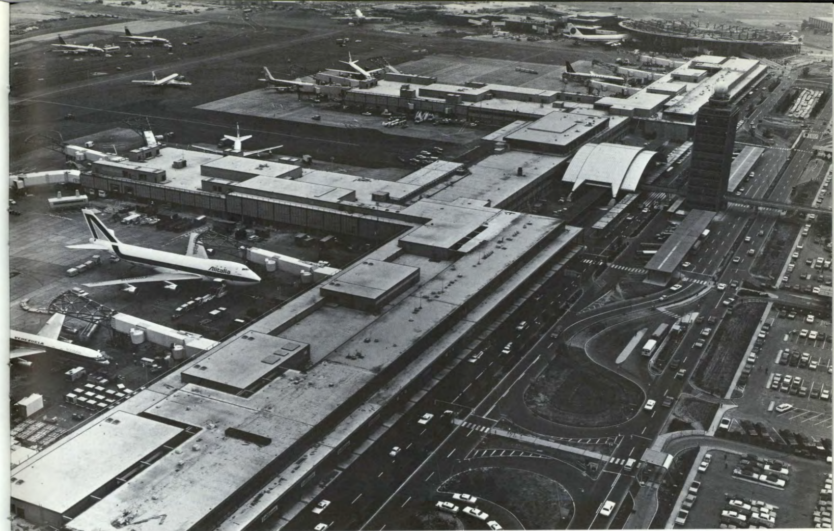
At John F. Kennedy International Airport, the aerial gateway of the United States, the International Arrival Building and Airline Wing Buildings complex was expanded to twice the original size at a cost of $65 million.
