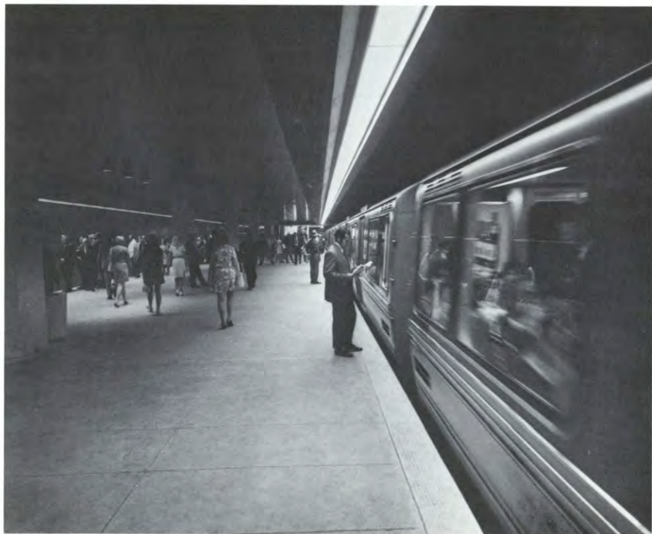
The spacious platforms (below) are more than 500 feet long, which will permit the operation of longer trains and thus provide greater passenger capacity and comfort.
