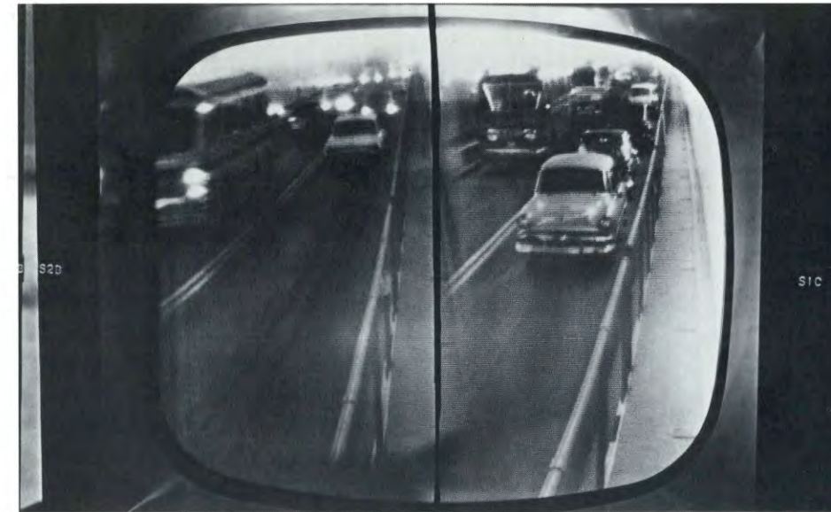
A split-screened TV monitor of the Tunnel Traffic Control System shows the approach to and departure from one of the numerous monitoring points.
