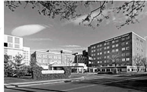
Exterior Somerset Medical Center
