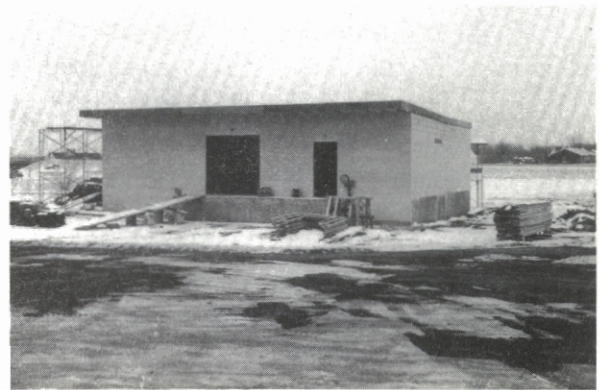
New paint storage building at Hightstown.
