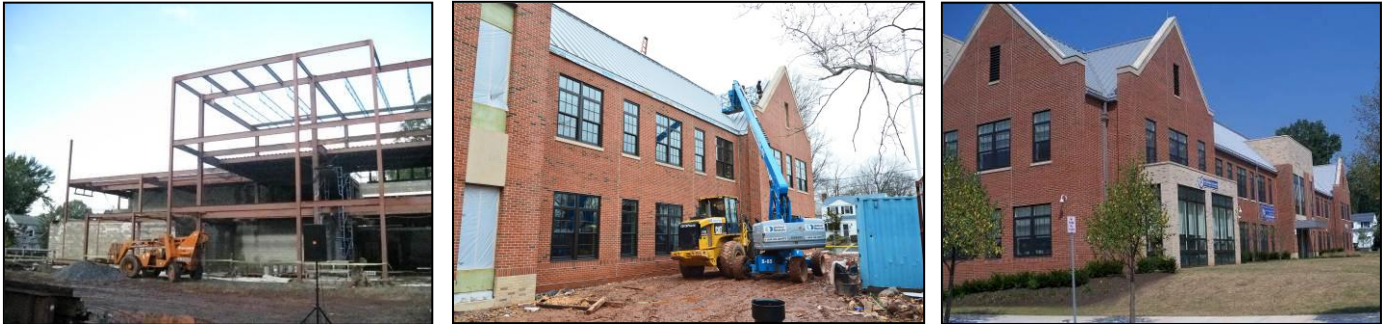
Construction of Victor Mravlag Elementary School
