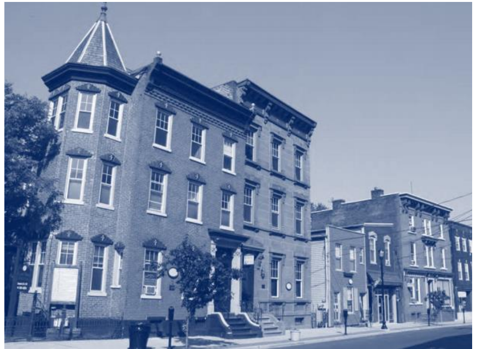
Phillipsburg, Warren County; Source: New Jersey Highlands Council
