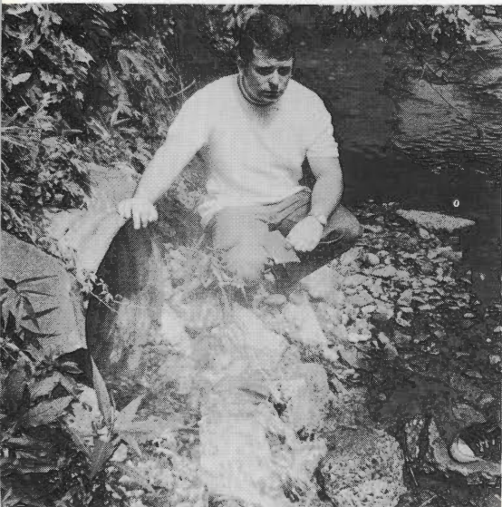
Left, inspecting a pipe discharging hot water, chemicals, steam, and fumes into the Elizabeth River
