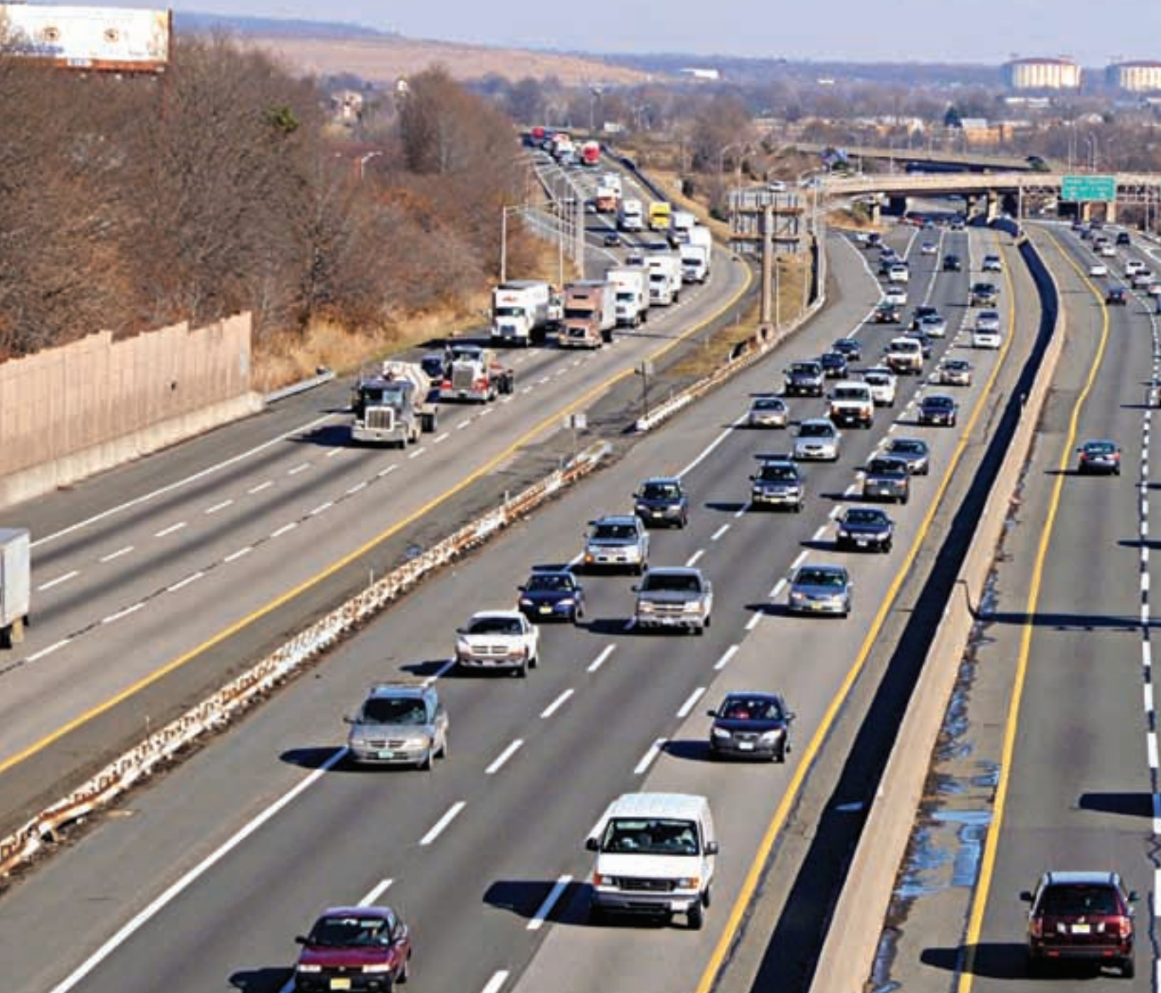
Cover photo: Construction of Hackensack River Bridge 1951 Above photo: NJ Turnpike mainline just south of Interchange 11
