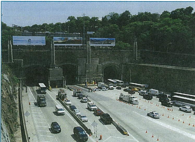
FIGURE 1-4: NEW JERSEY PORTALS OF THE LINCOLN TUNNEL
