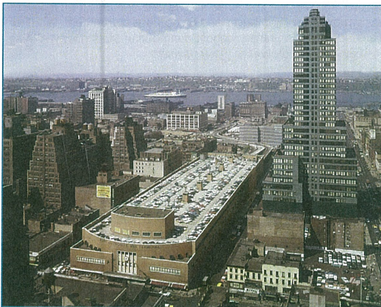
FIGURE 1-5: PORT AUTHORITY BUS TERMINAL OPENED IN 1950
