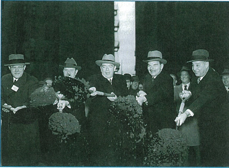
FIGURE 1-3: GROUNDBREAKING OF THE BUS TERMINAL
