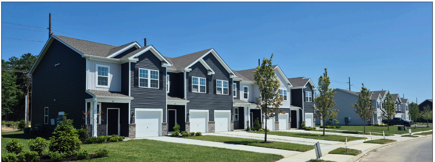
Above: Ocean Club in Egg Harbor Township, Atlantic County, redeemed a total of 20.75 PDCs for the development of 657 dwellings. Photo/Paul Leakan
