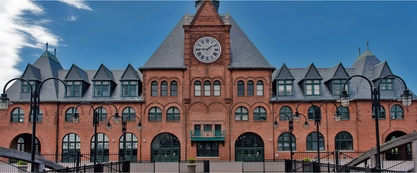
Above photo: The historic Central Railroad of New Jersey (CRRNJ) Terminal in Liberty State Park, Jersey City.
