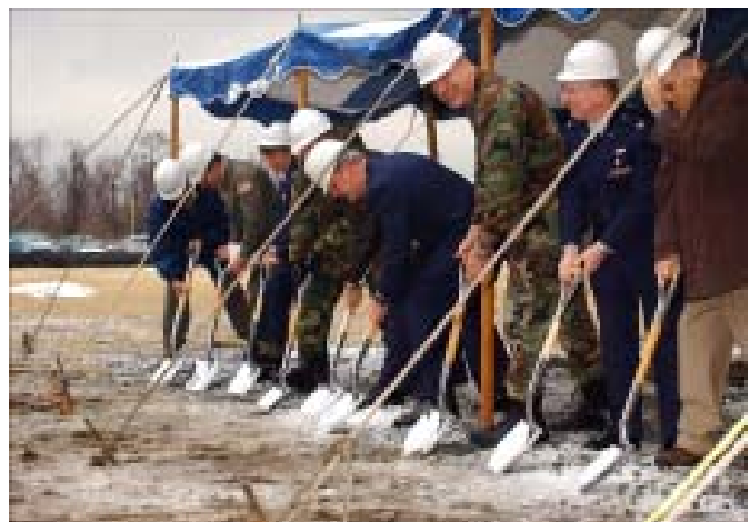
Col. (Ret.) Aldo Baldi (far right), former 108th Medical Squadron Commander joins members of the Guard, Reserve and active-duty Air Force in breaking ground on the new Joint Medical Training Facility at McGuire Air Force Base on March 6. Col. Baldi conceived the concept for the Facility 10 years ago.
