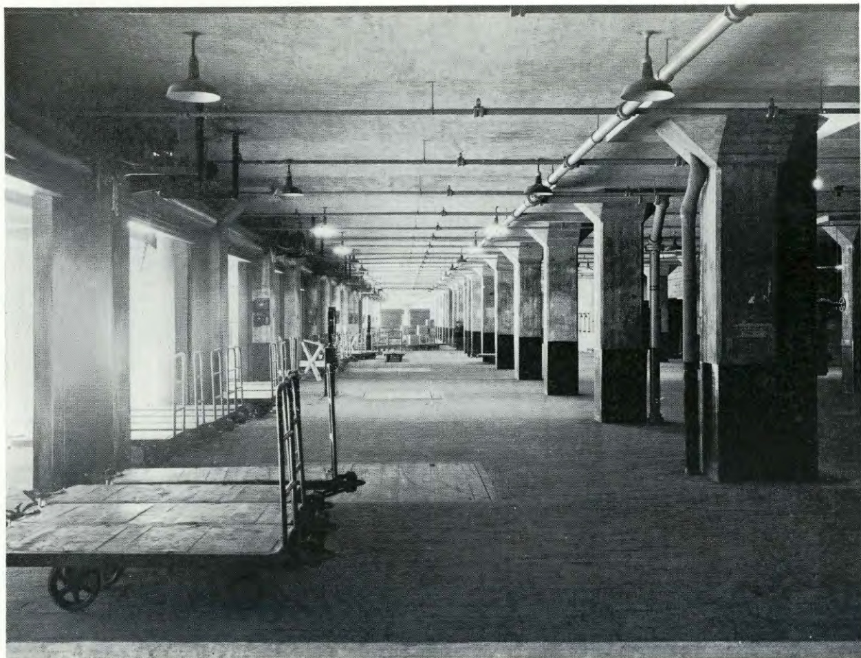
Port Authority Commerce Building, Interior View of Union Inland Freight Station
