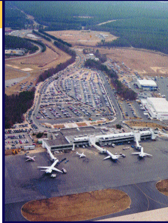
Terminal Area, Atlantic City International Airport. General Aviation Ramp is on right
