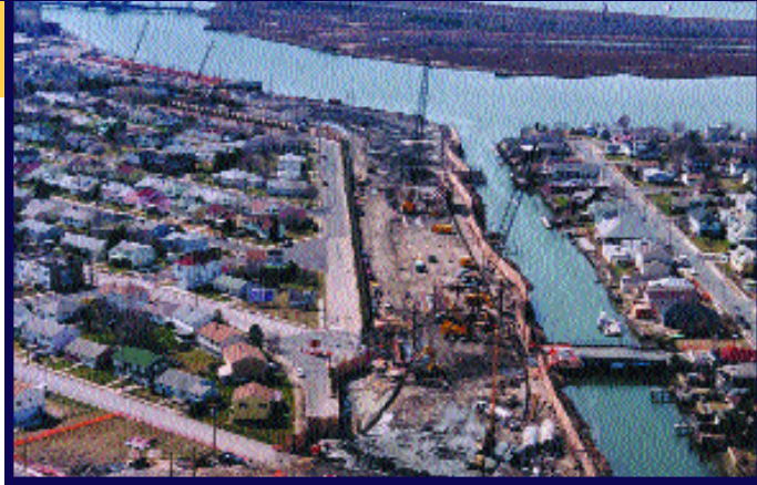
Atlantic City / Brigantine Connector Project, early construction phase along Penrose Canal
