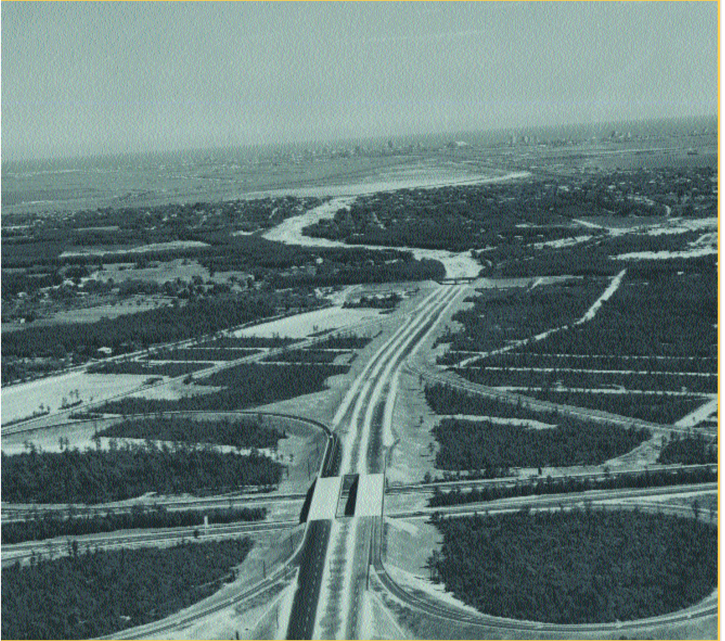
Parkway Interchange, 1964. An aerial view of the clover leaf adjoining the Atlantic City Expressway to the Garden State Parkway.
