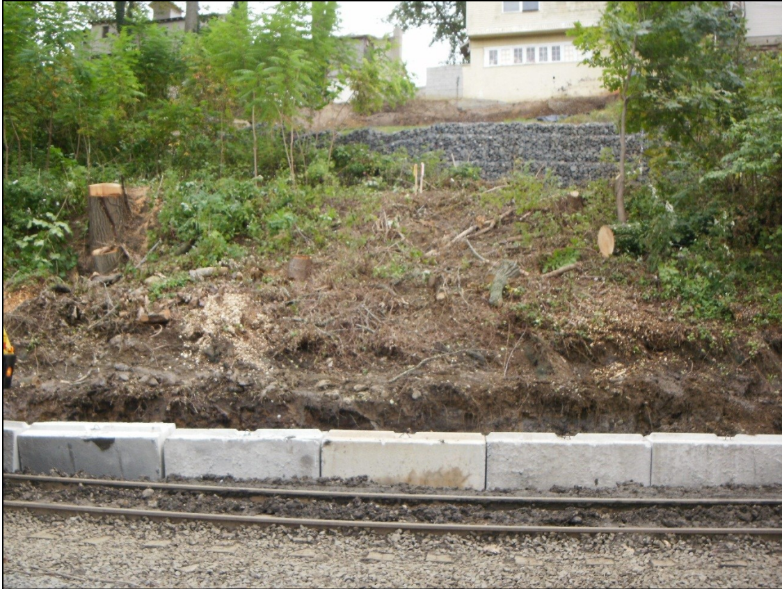
Temporary protection – post Hurricane Irene
