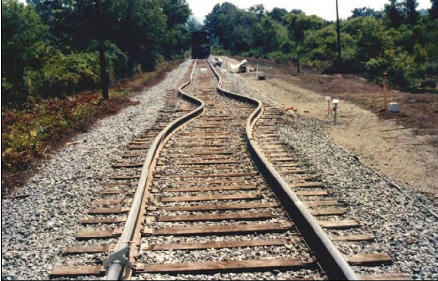
Rail Buckled from High Heat 12 - Photo Courtesy of USDOT Volpe Center
