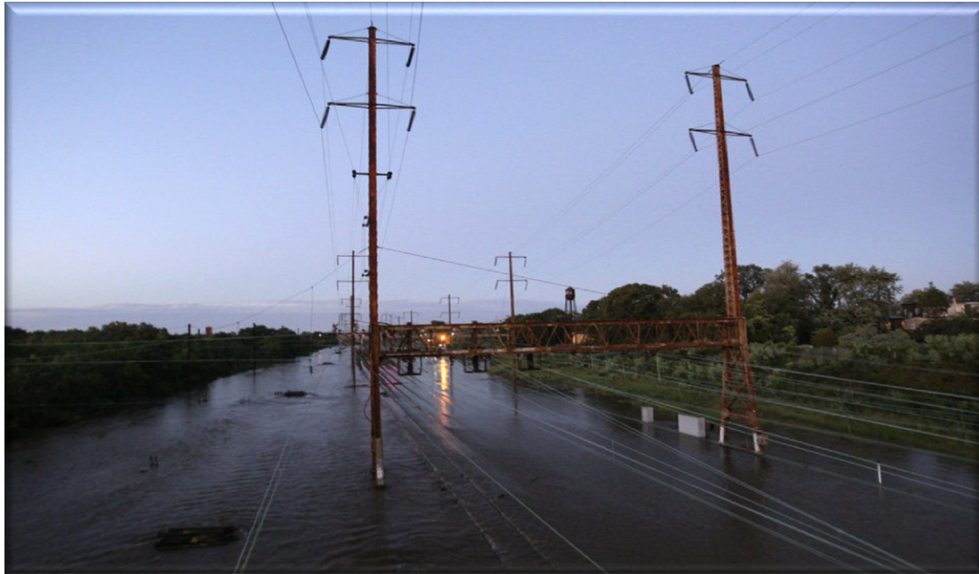
Northeast Corridor Flooding from Hurricane Irene
