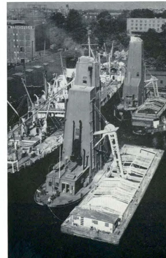
Six floating grain elevators, capable of transferring grain between ships, barges and shore installations, were purchased by the Port Authority early in 1958 to assure their continued service and availability to shippers in the New Jersey-New York Port.
