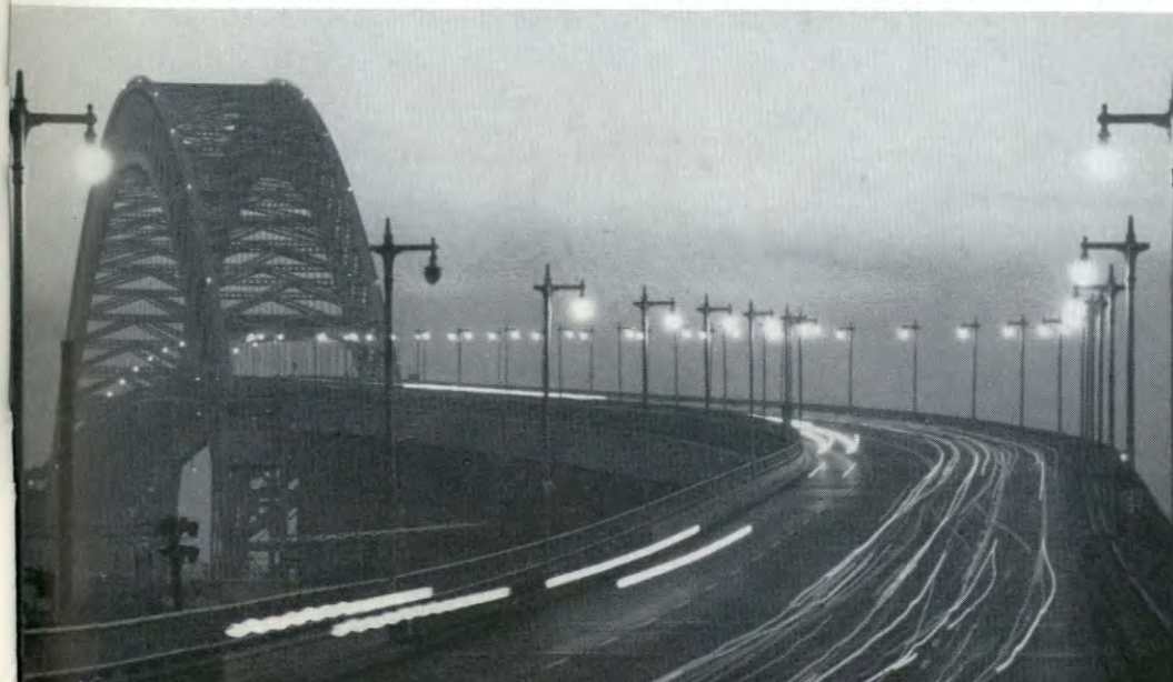
Steel arch Bayonne Bridge spans the Kill Van Kull between Bayonne, New Jersey and Staten Island, New York.
