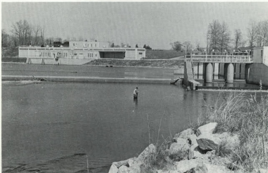
Pumping station at Hamden where water is drawn from the South Branch for Round Valley Reservoir
