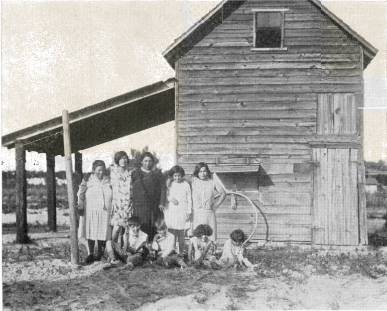
This house started out as a barn. It does not seem suitable for housing people
