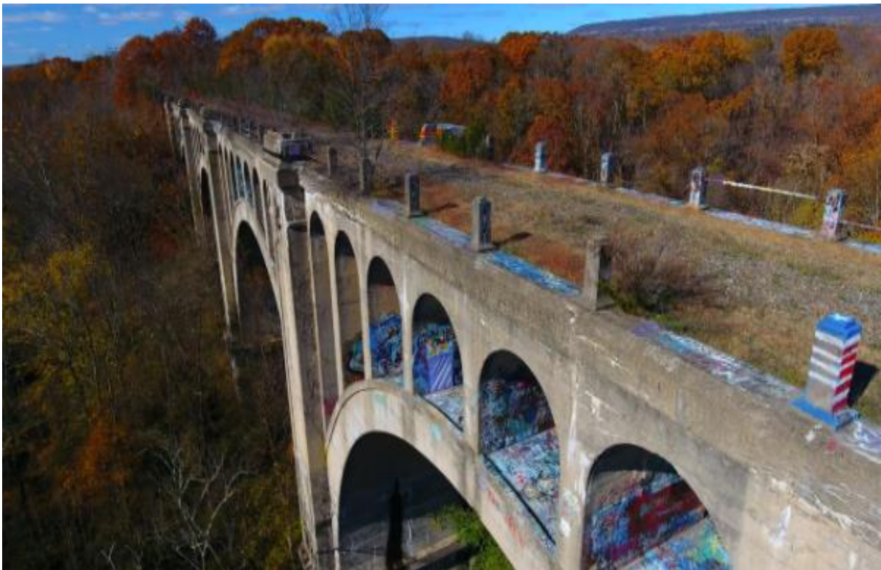
Paulinskill Viaduct (Source: Lehigh Valley Live)
