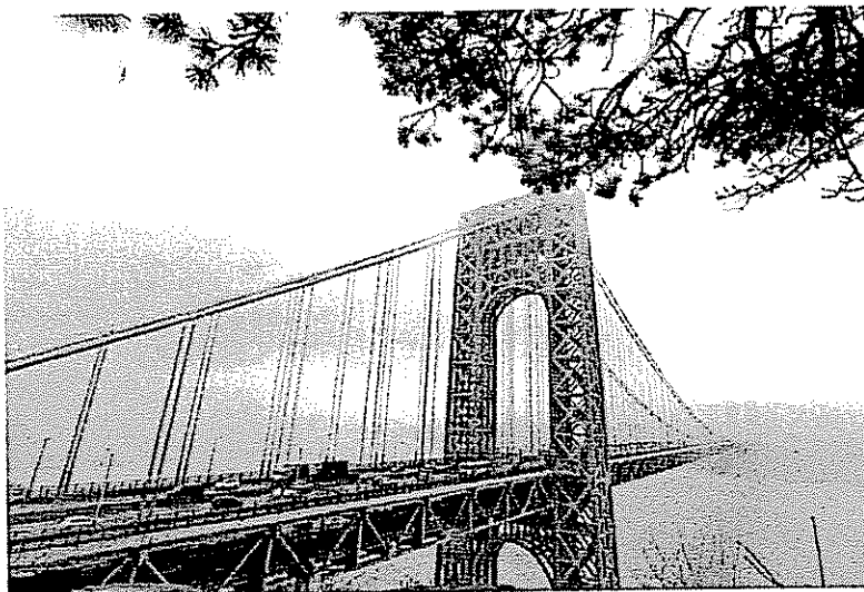
The George Washington Bridge.
