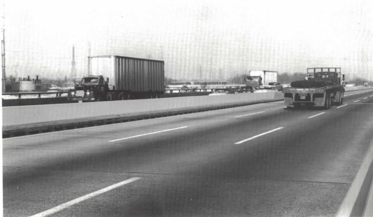
Median concrete center barrier installed on Raritan River Bridge near New Brunswick.
