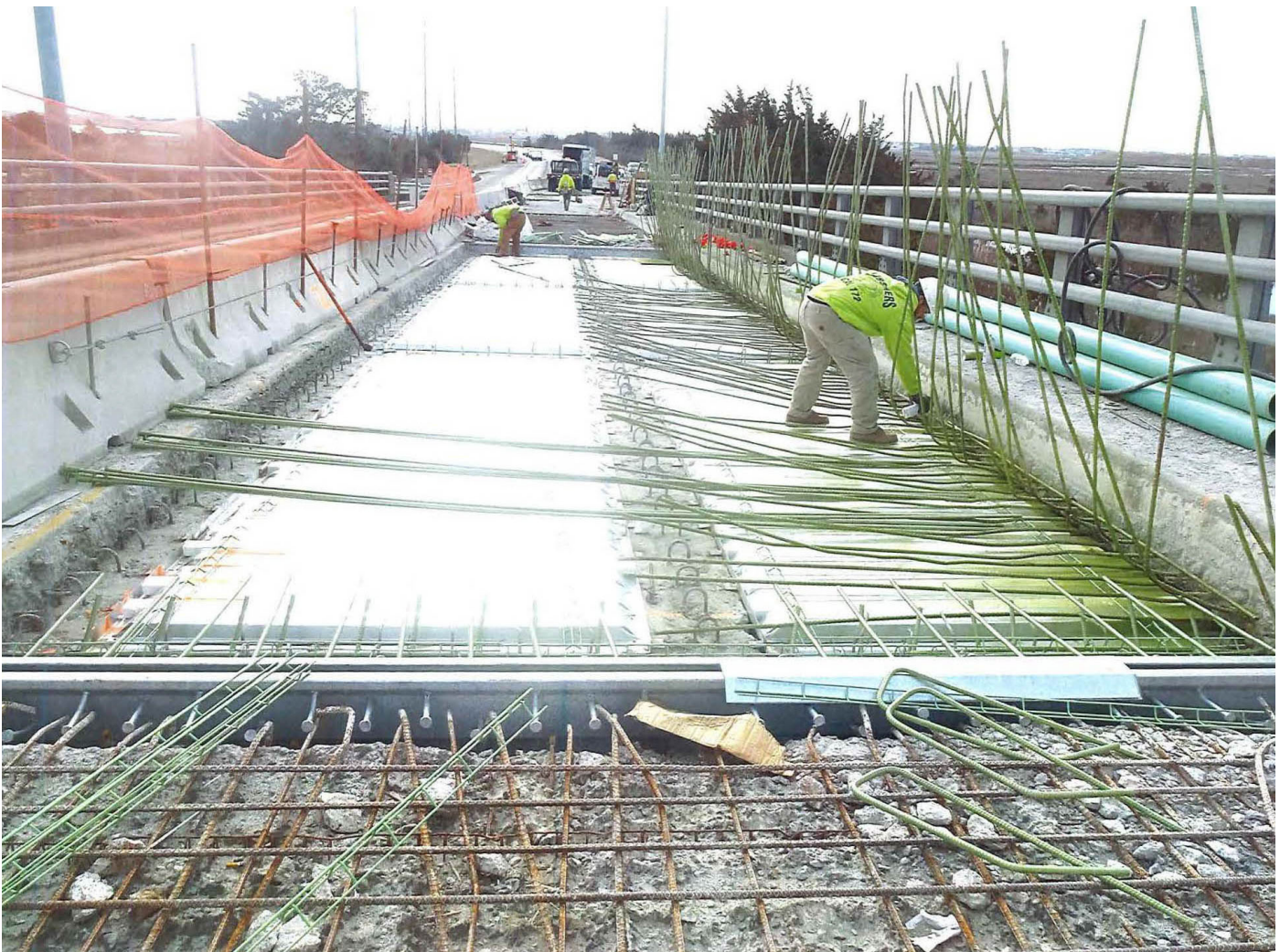
Cape May County Avalon Boulevard Bridge Deck Rehabilitation. SFY2022 Loan: $9,627,220.
