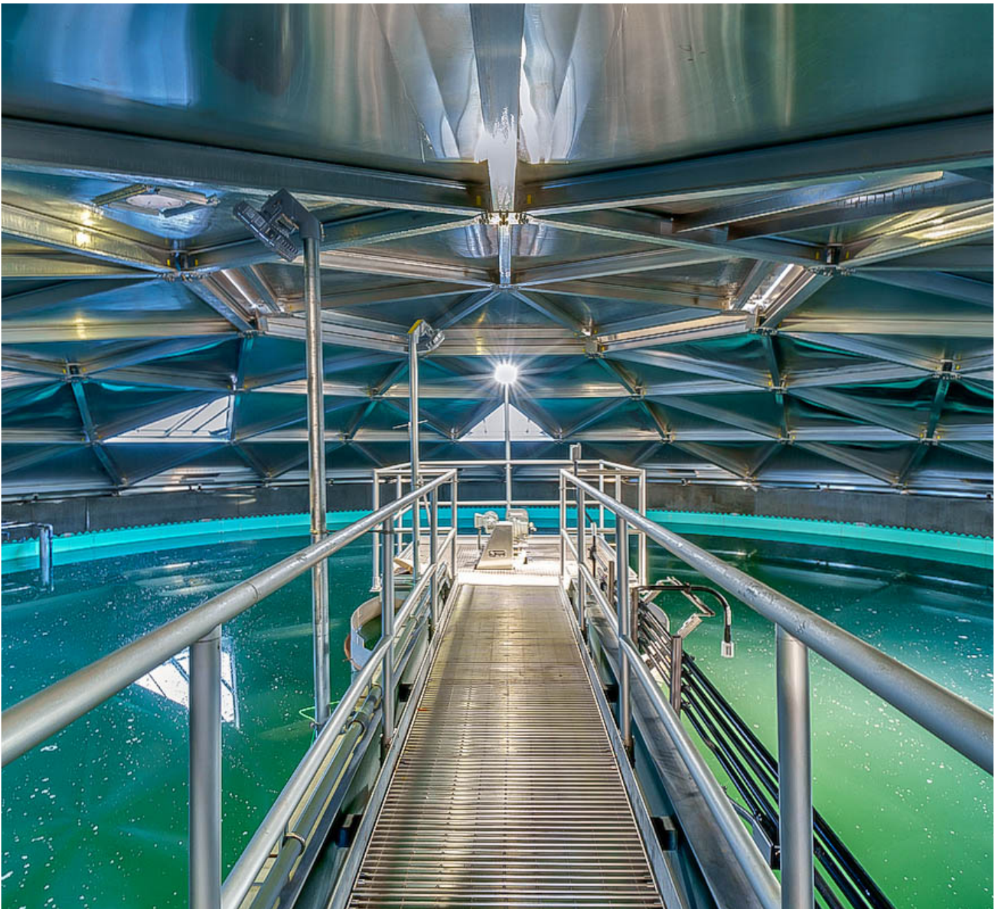
Somerset Raritan Valley SA WWP Rehab Improvements. SFY2022 Loan $5,547,220
