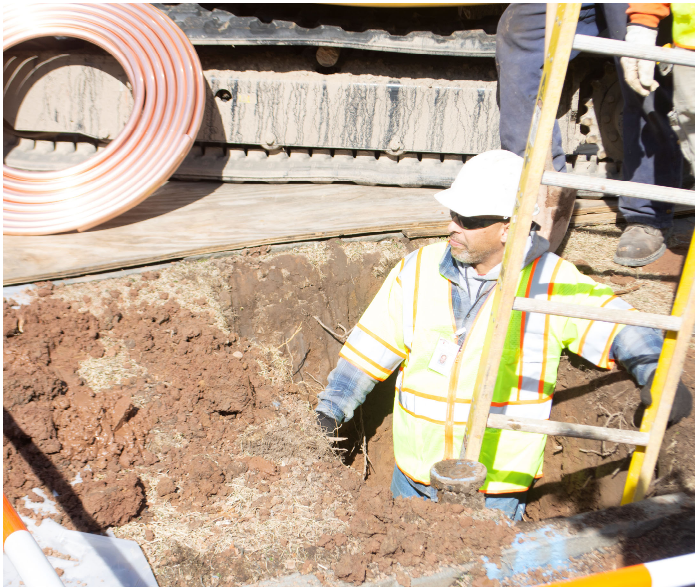
Newark City Lead Service Line Replacement. SFY2022 Loan: $89,203,472
