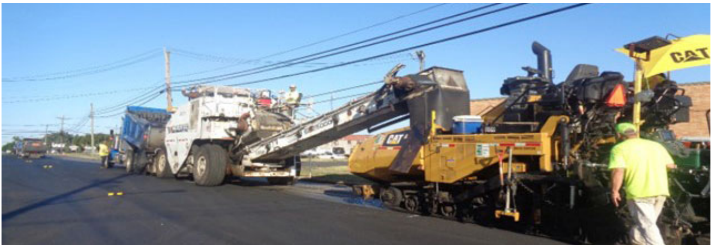
Camden County Westfield Avenue Reconstruction. SFY2022 Loan: $1,786,364
