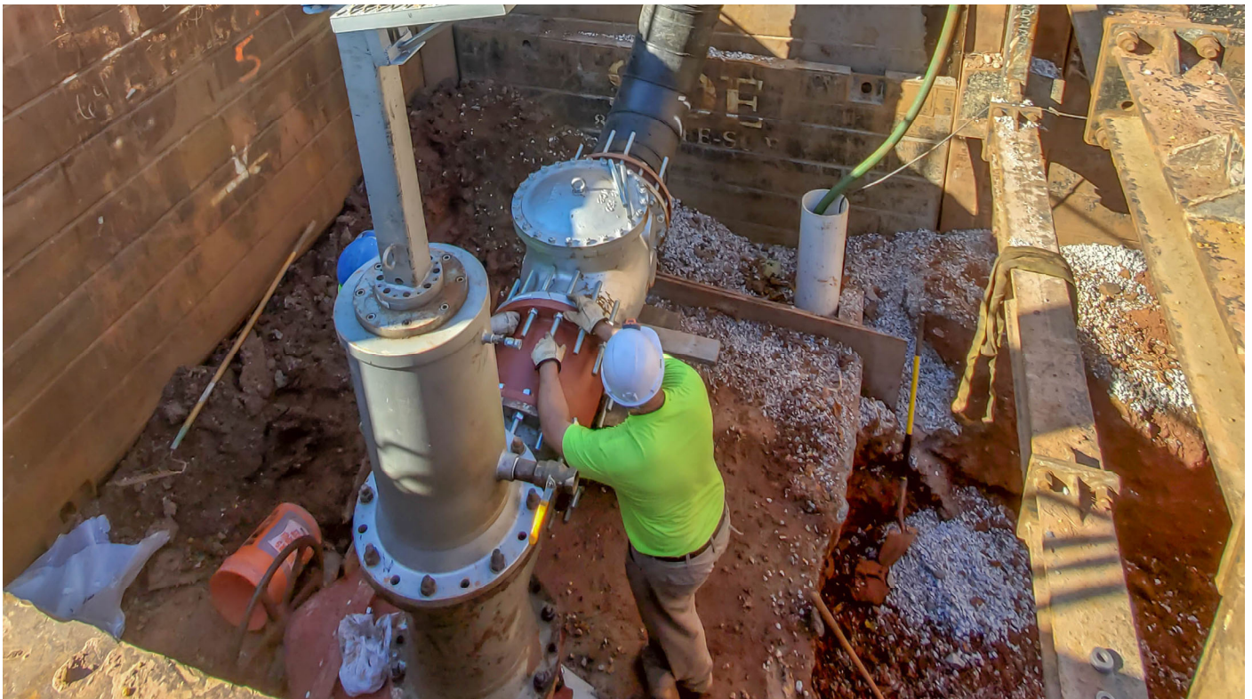
Carteret Borough Roosevelt & Bergen Street Pump Station Upgrades. SFY2022 Loan: $5,398,616.
