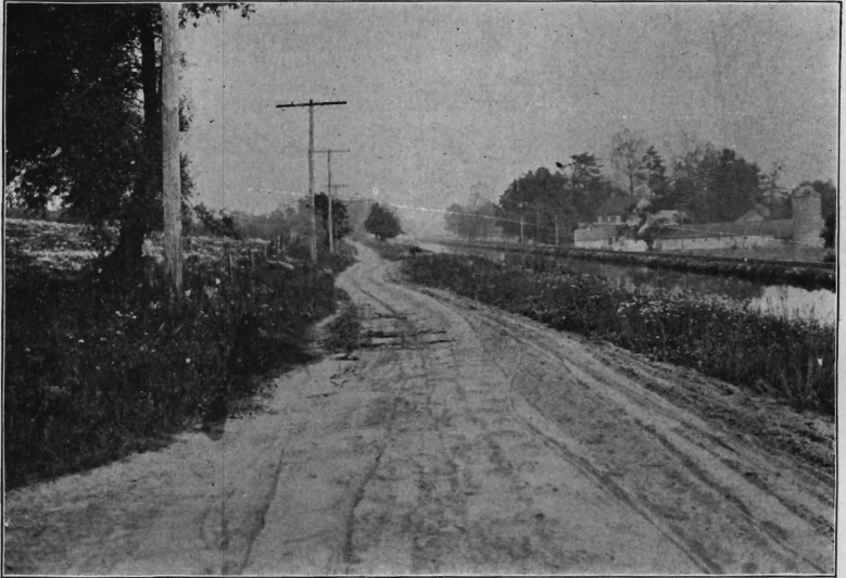
Upper River Road, Mercer County, Before Improvement
