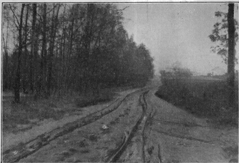
Berlin and Milford Road, Camden County, Before Improvement
