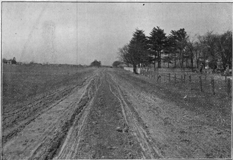
Port Reading Railroad Road, Middlesex County, Before Improvement
