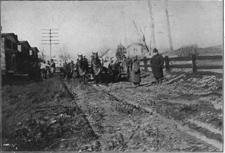
Haddonfield Hill, Camden County, Before Improvement, Showing Intersection of Ellis and Potter Streets
