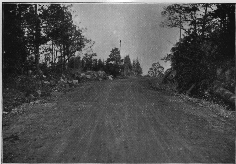
Midvale Road, Passaic County, After Improvement
