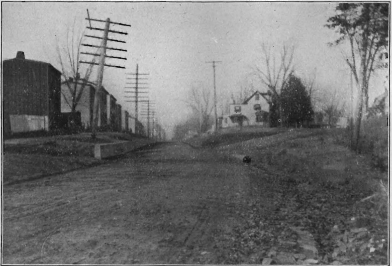
Haddonfield Hill, Camden County, After Improvement, Showing Concrete Retaining Wall on Ellis Street with Stone Gutters to the bottom of the hill
