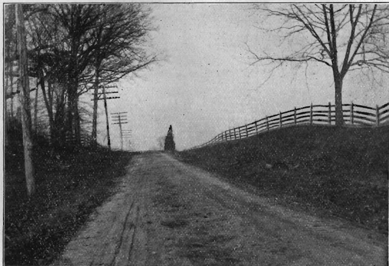
Haddonfield and Coffin's Corner, Camden County, Kay's Hill Before Improvement
