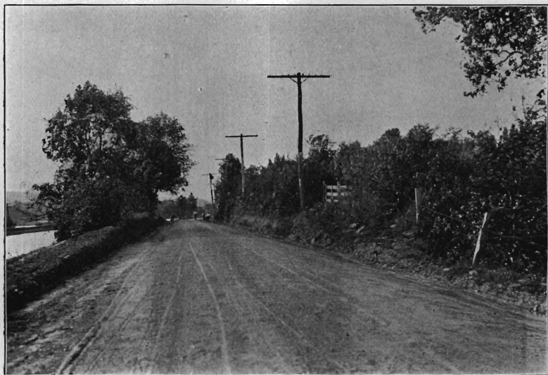
Upper River Road, Mercer County, After Improvement
