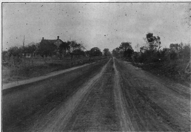
Goshen Road, Cape May County, After Improvement
