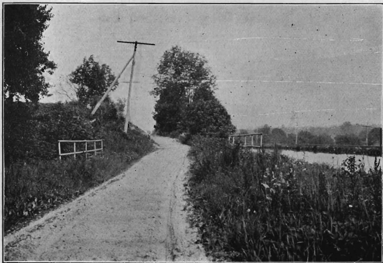
Upper River Road, Mercer County, Before Improvement
