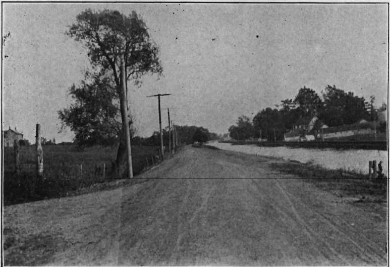
Upper River Road, Mercer County, After Improvement
