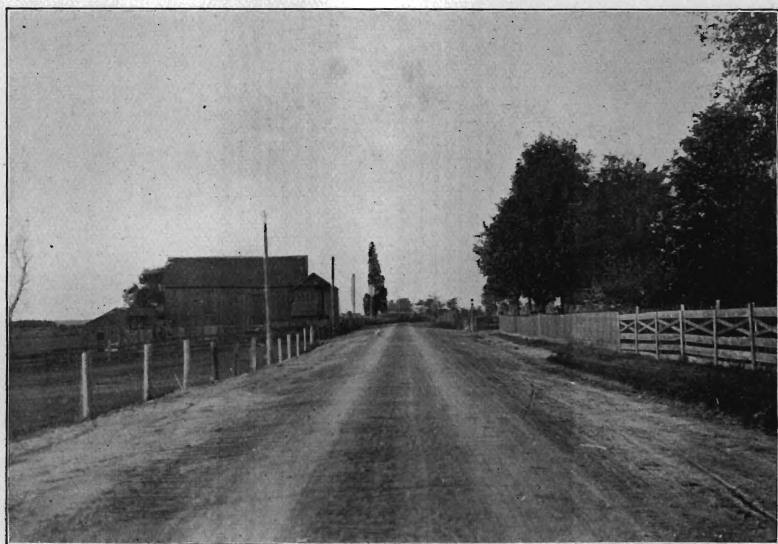
Quaker Bridge Road, Mercer County, After Improvement
