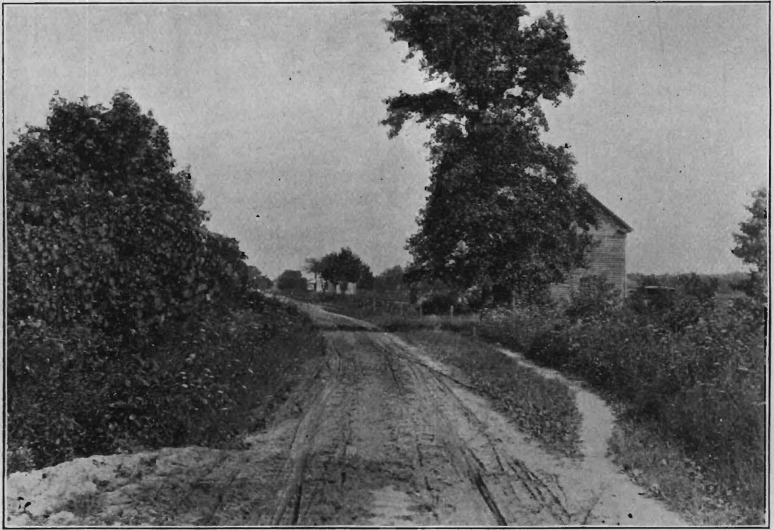
Goshen Road, Cape May County, Before Improvement
