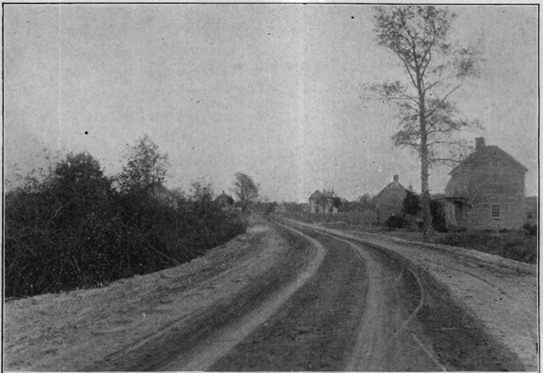
Goshen Road, Cape May County, After Improvement
