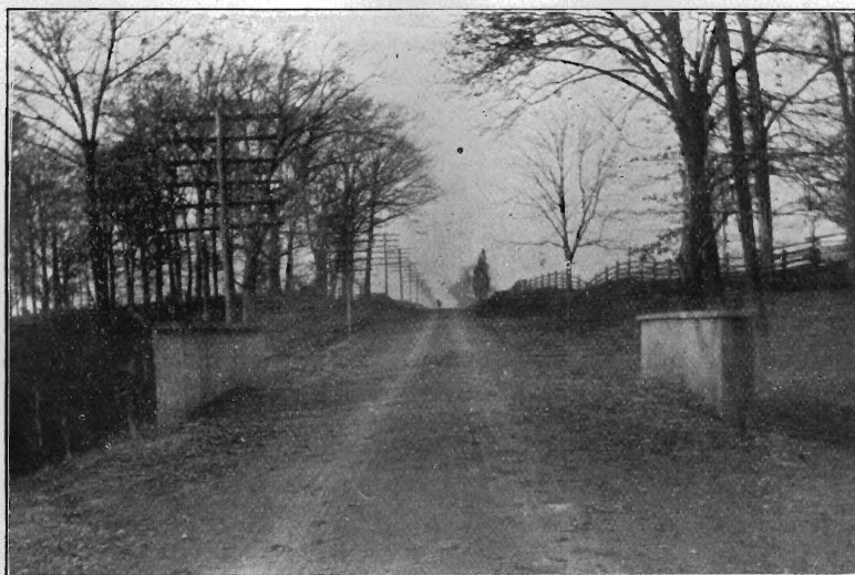
Haddonfield and Coffin's Corner, Camden County, Kay's Hill After Improvement Showing Concrete Bridge
