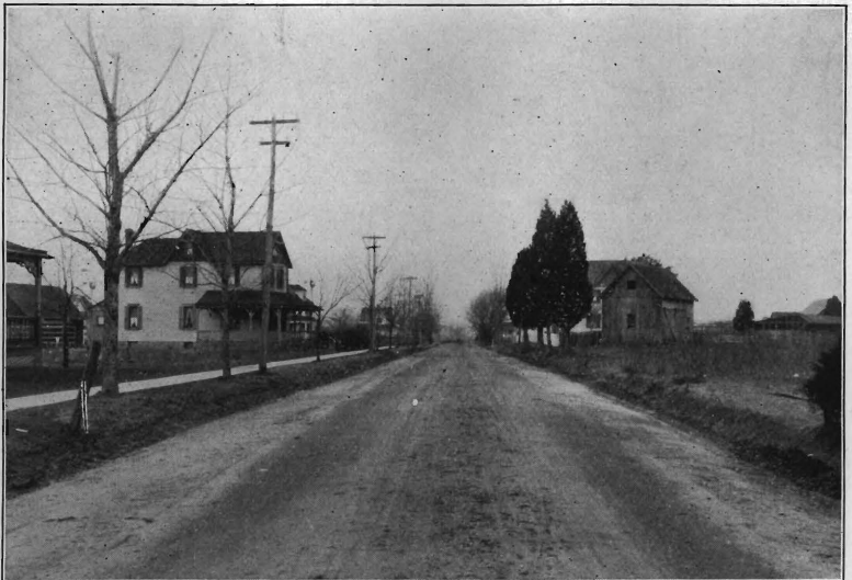
Linden Avenue, Laurel Springs, Camden County, After Improvement
