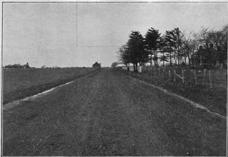
Port Reading Railroad Road, Middlesex County, After Improvement
