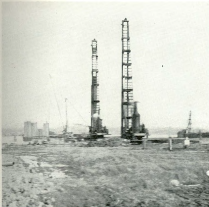
Driving sheet piling around crib at Perth Amboy end, Outerbridge Crossing.
