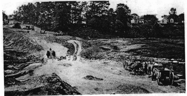
Highway Construction Early 1900s
