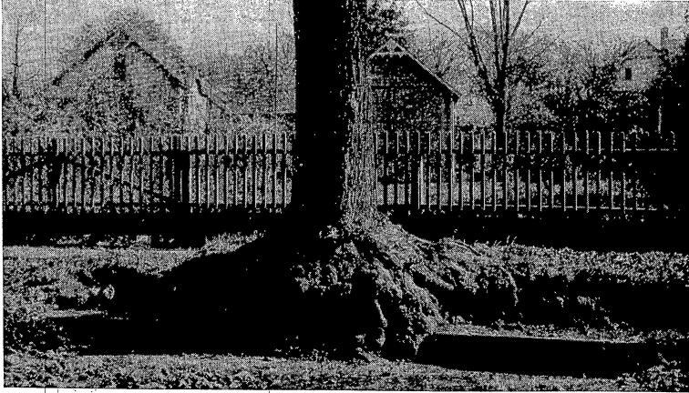
Fig. 9. Such exposure of roots is bad, but may be tolerated until a new tree can be established.
