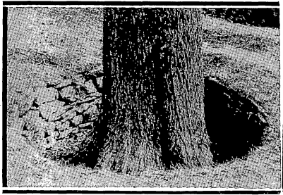
Fig. 24. A "Well" constructed about an elm tree when grade was raised. Photo by Wm. Solotaroff.
