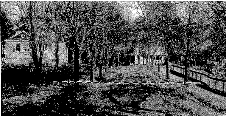
Fig. 25. Street grade raised two feet without changing sidewalk or injuring trees. Practicable only on a side street.
