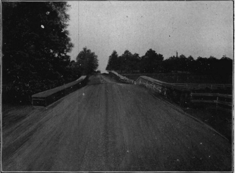
White Horse Road, Mercer county, entering Trenton, 4-inch macadam, bearing heavy traffic.
