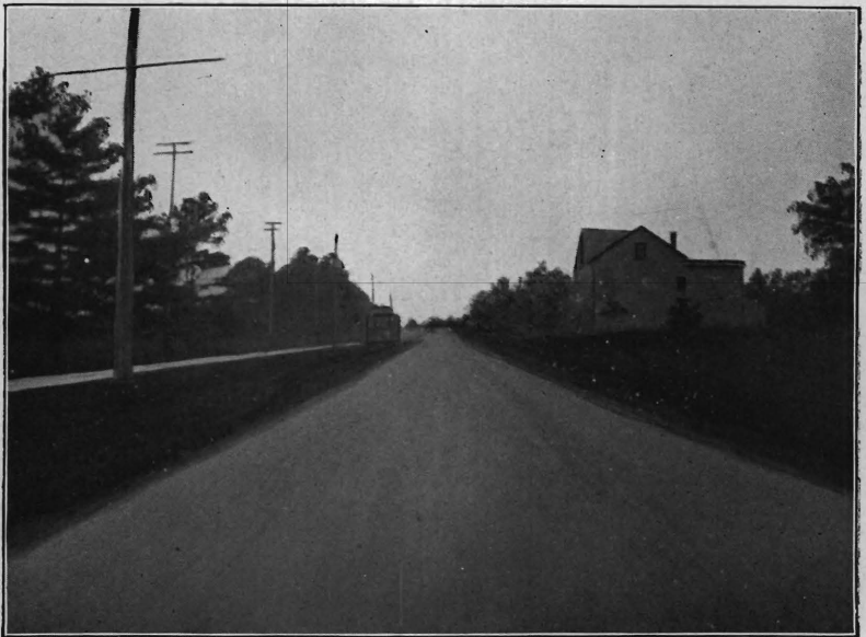
Pennington and Trenton Road, Mercer county, 6 and 8-inch macadam, bearing heavy traffic.
