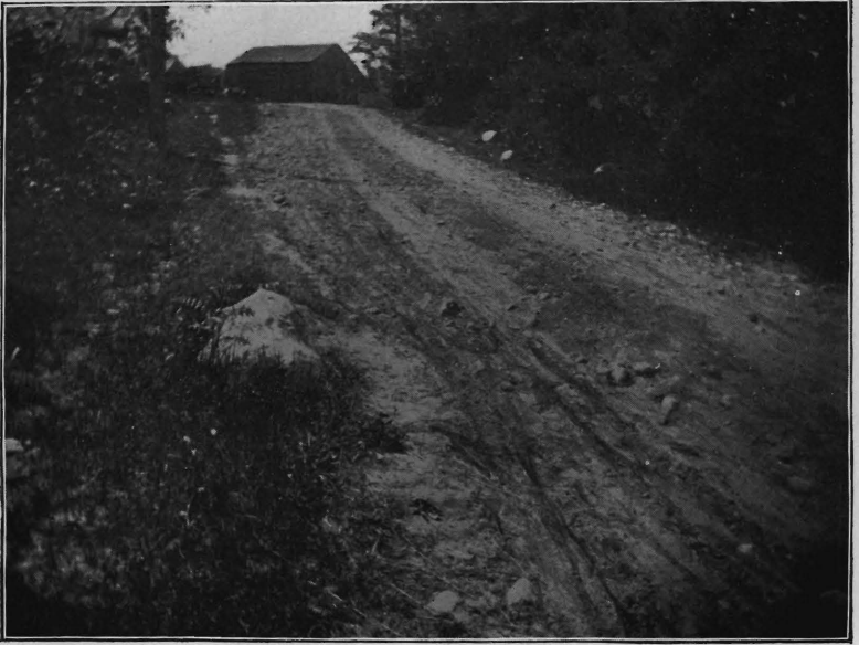
Denville and Pine Brook, Morris county. Before.
