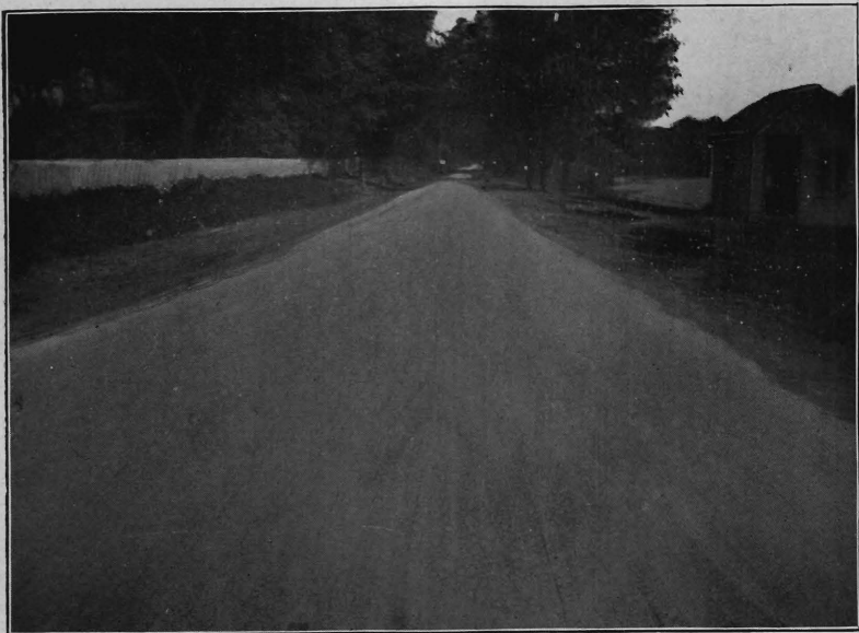
Mine Brook Road, Somerset county, rock bottom, 6 inches thick, surface 4 inches thick. -
