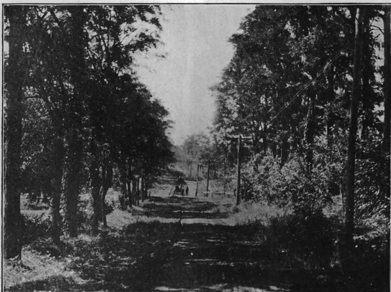
Navesink and Hillside Road, Monmouth county. Before improvement.
