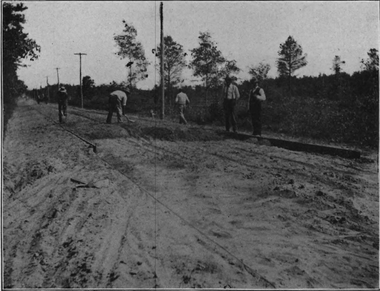
Franklinville Road, Gloucester county. Laying Gravel bed over sand.
