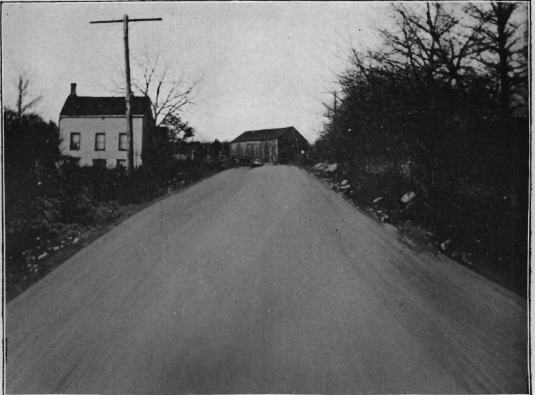
Denville and Pine Brook, Morris county. After. 6-inch macadam.
