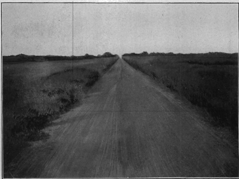
May's Landing and Egg Harbor City Road, Atlantic county. Gravel over heavy bed of sand.
