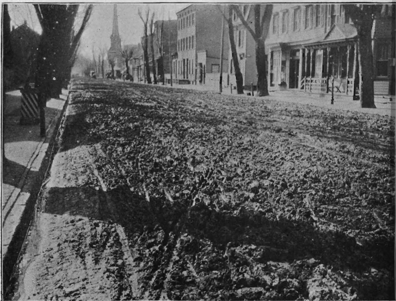
Farnsworth Avenue, Bordentown, Burlington county. Before improvement.
