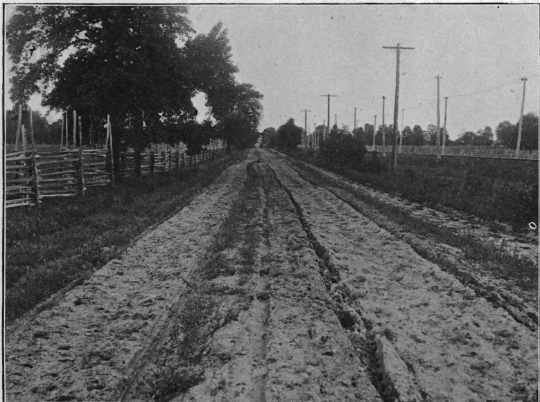
Burlington and Mt. Holly Road, Burlington county. Before. Sand and clay bottom.
