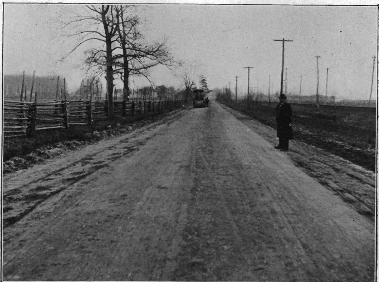
Burlington and Mt. Holly Road, Burlington county. After. 6-inch macadam, 14 feet wide.
