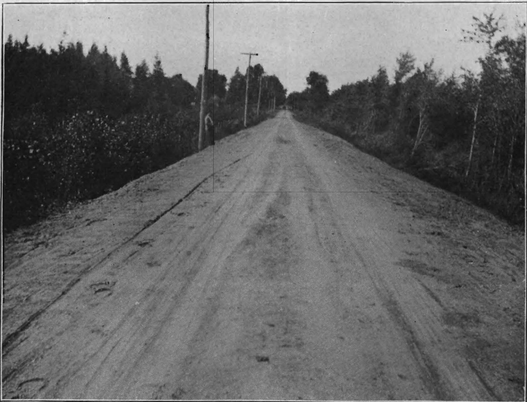
Franklinville Road, Gloucester county. After gravelling.
