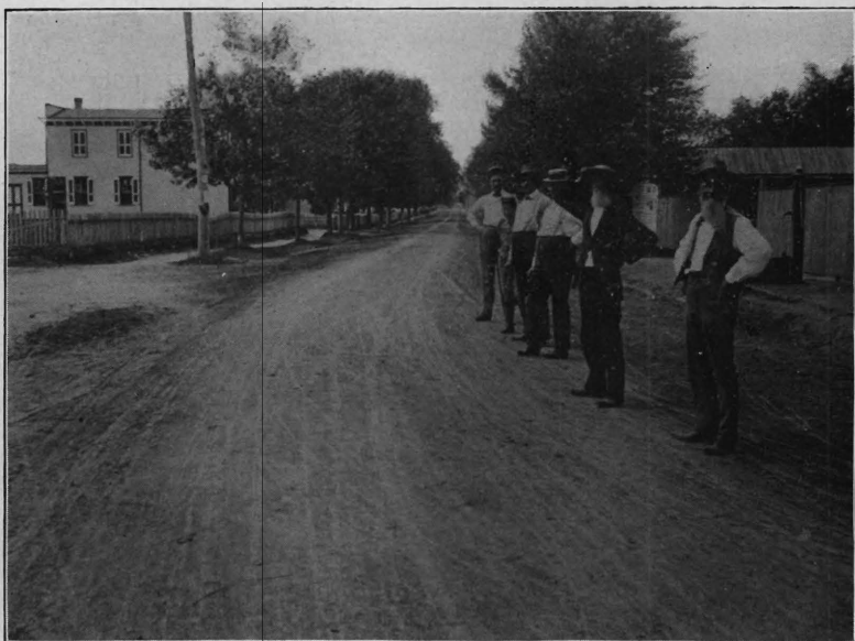
Franklinville Road, Gloucester county. After improvement. Gravel.
