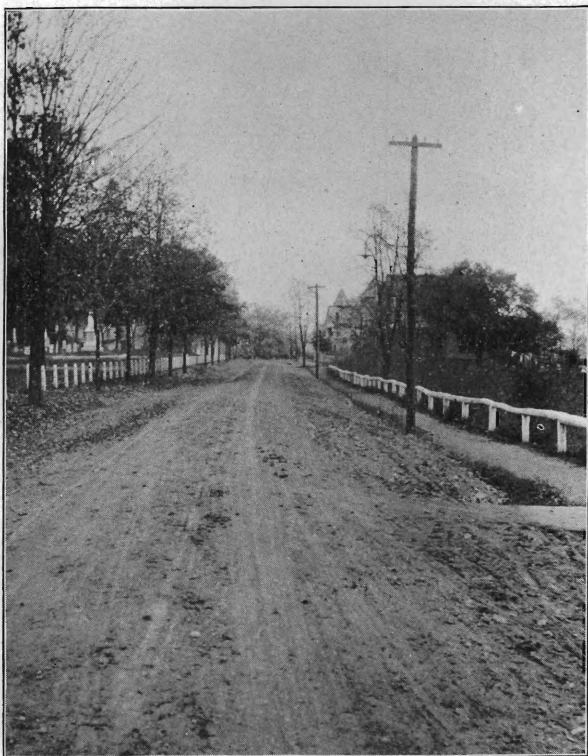
Finished Bed, Watchung Avenue, Essex county, boulder, telford bottom 5 inches, macadam surface 3 inches,
