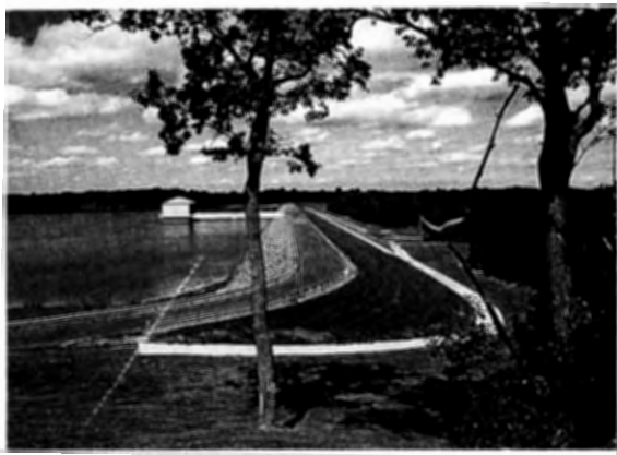
The Main Dam of the Manasquan Reservoir creates a 770 acre Reservoir in the Timber Swamp Brook in Howell Township, Monmouth County.
