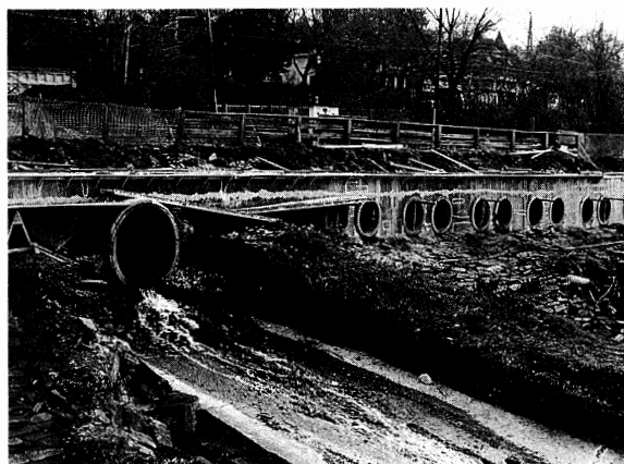
The rehabilitation of the Washington Crossing waste gate and spillway in Hopewell Township, Mercer County.
