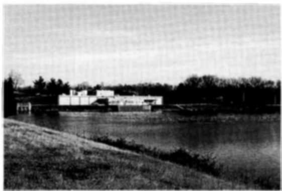
The South Branch Pump Station at Hamden, Hunterdon County maintains storage in Round Valley Reservoir by pumping surplus water from the South Branch of the Raritan River.
