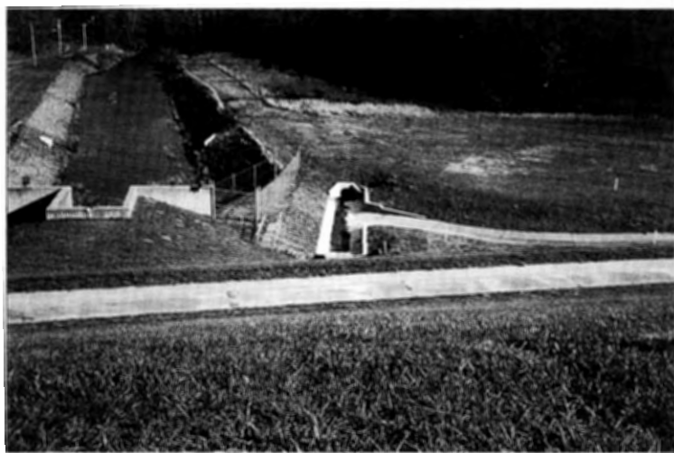
The Toe Drain Weir Channel Rehabilitation is one of several capital improvement projects completed at the Manasquan Reservoir Complex during 1999.
