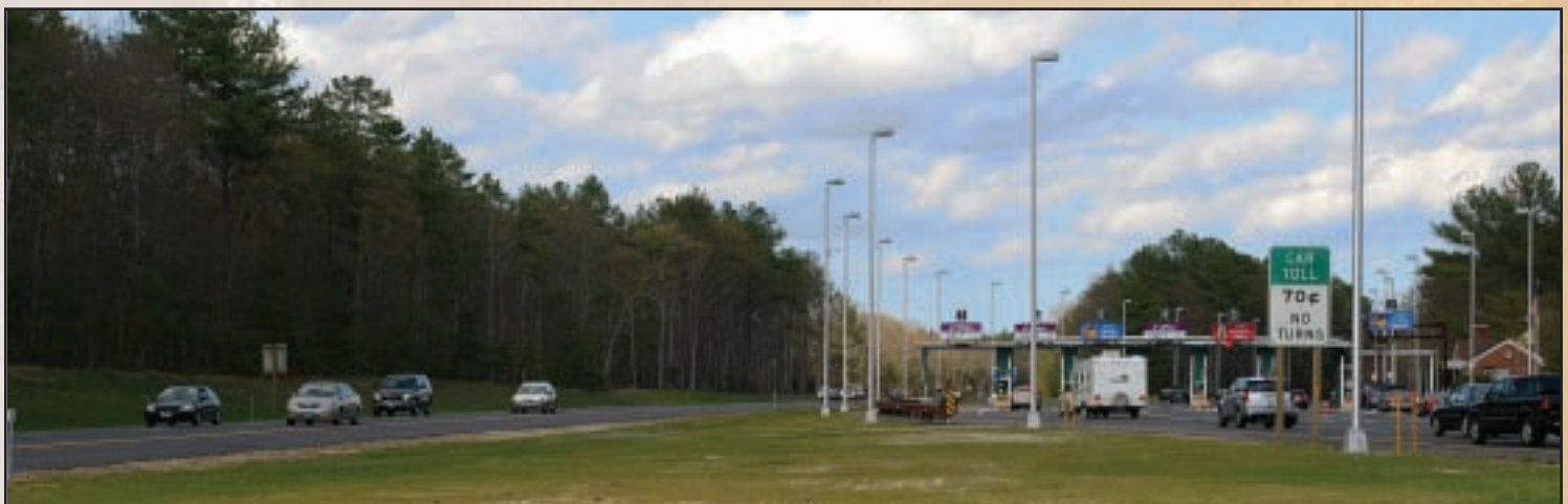
One-way tolling, Garden State Parkway, New Gretna Toll Plaza
