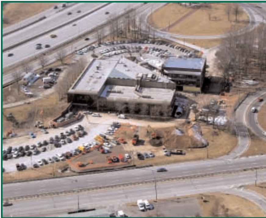
Overhead view of TMC under construction
