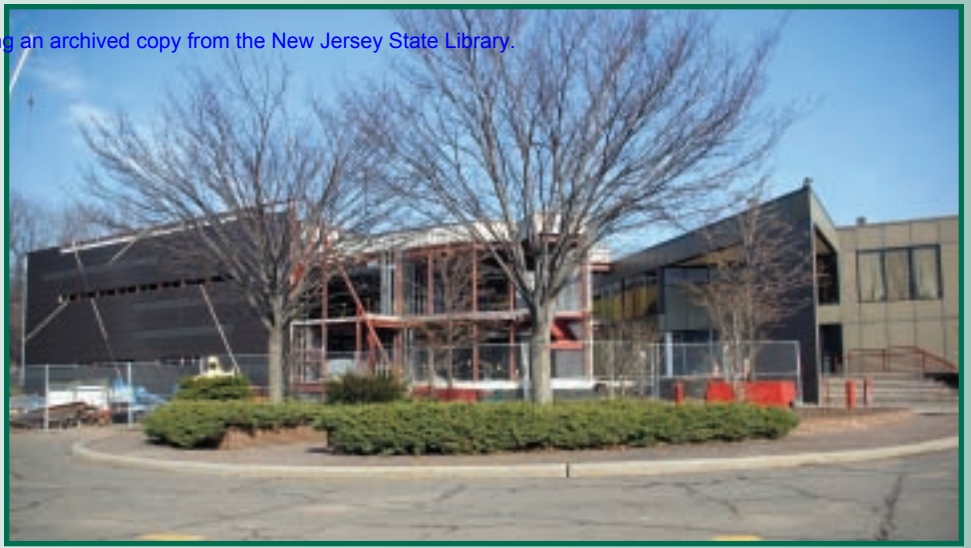
Traffic Management Center (TMC) under construction
