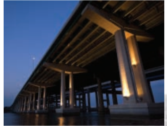
Underneath the Driscoll Bridge
