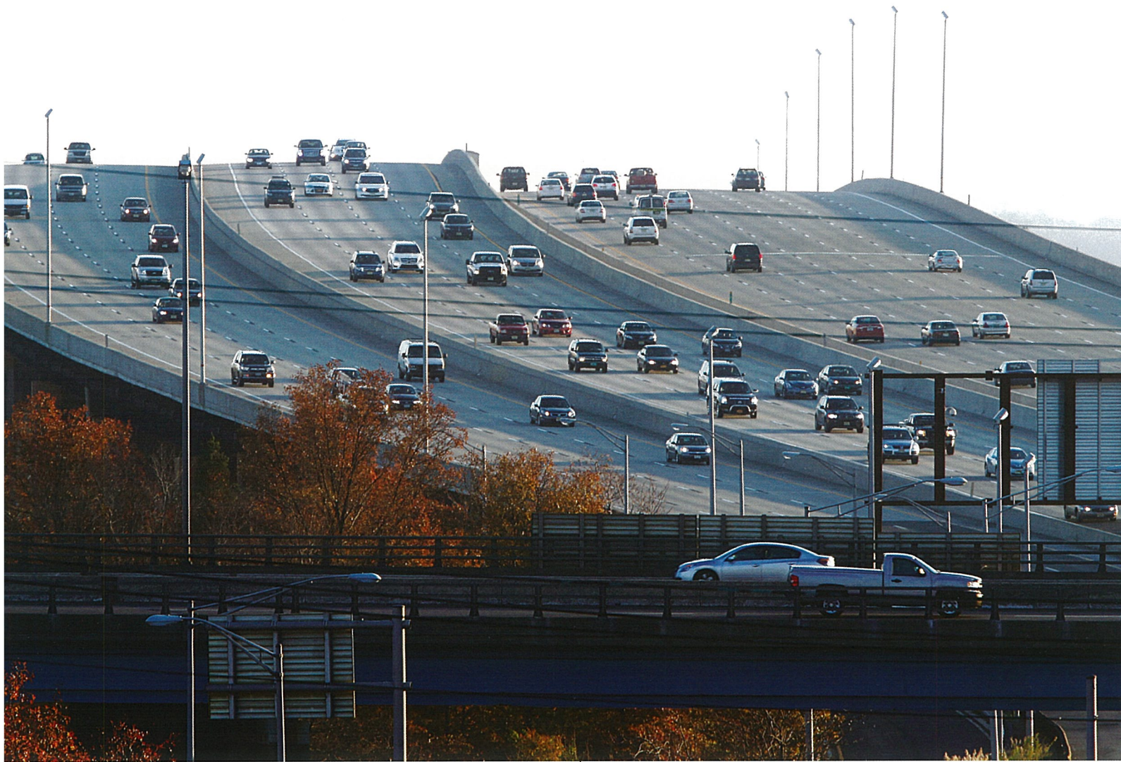
Driscoll Bridge on the Garden State Parkway, Middlesex County.
