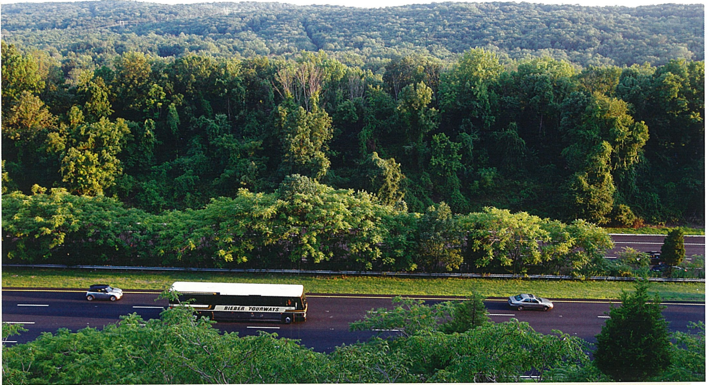
Interstate 78, Bridgewater, Somerset County.
