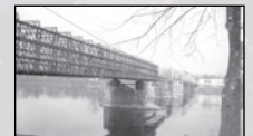
Yardley-Wilburtha Bridge taken out of service; 3 of its 6 spans lost in 1955 flood May 3, 1961
