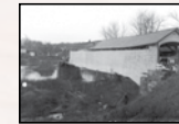
Portland-Columbia Toll Bridge opens; old covered timber bridge closed to vehicles December 1, 1953
