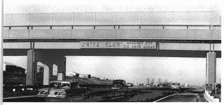
New panels installed on bridge piers to reflect color at night and keep motorists awake.
