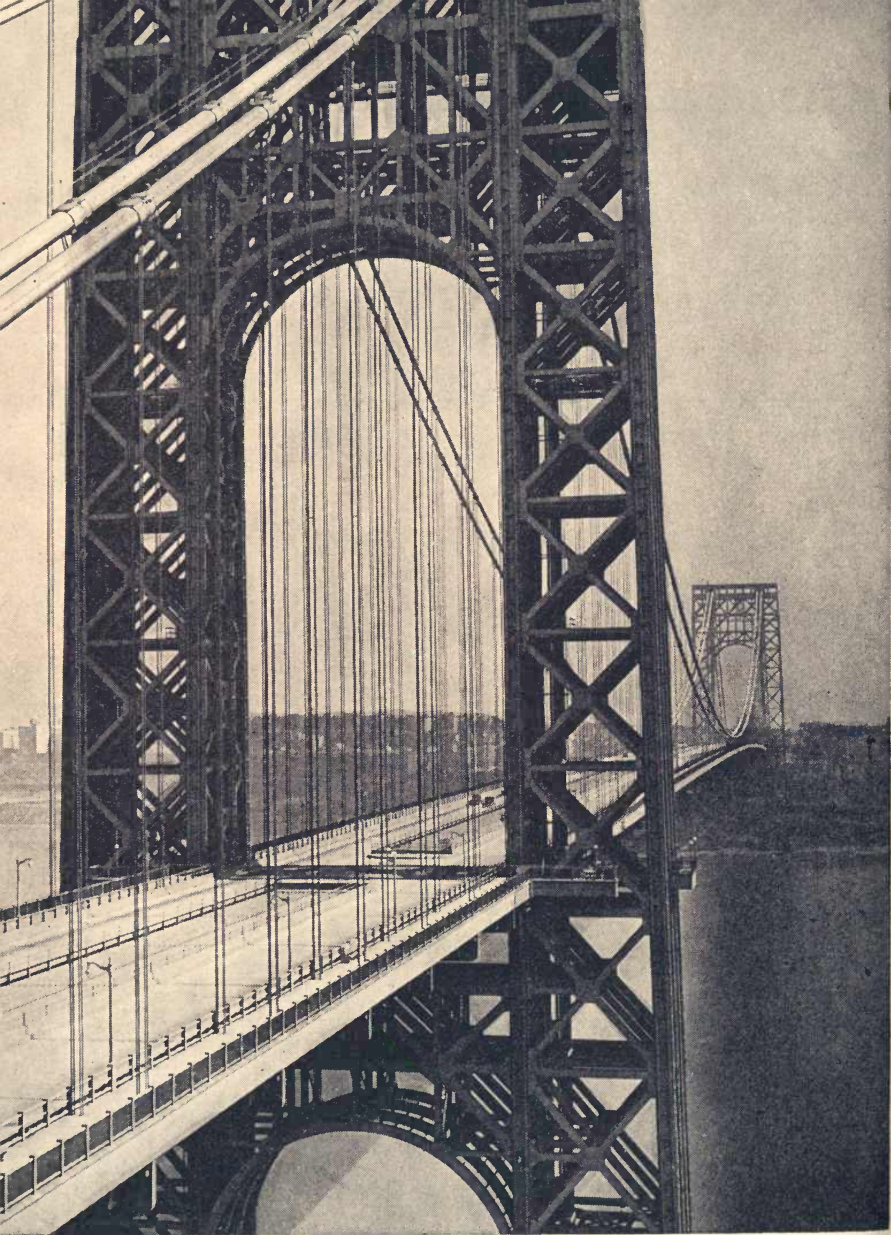
GEORGE WASHINGTON MEMORIAL BRIDGE
