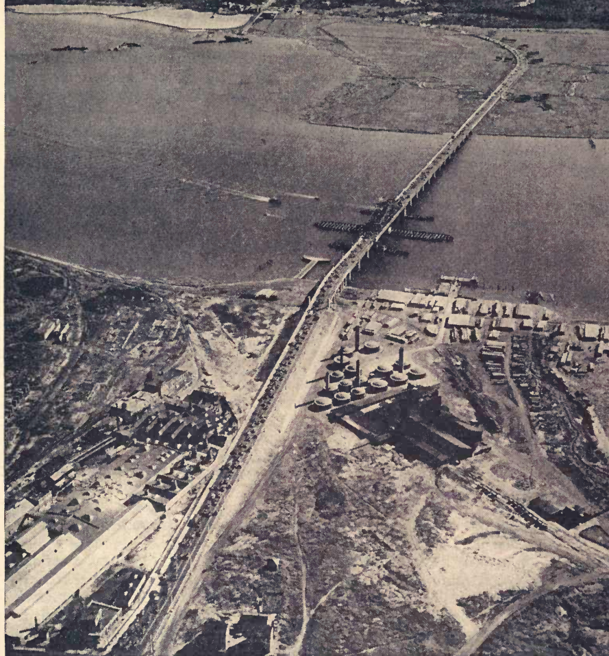
THE RARITAN RIVER AT PERTH AMBOY
