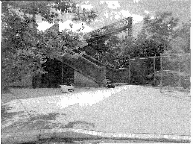
16. TRASH NEAR FOOT BRIDGE AT 7 TH AVE & NO 14 TH ST
