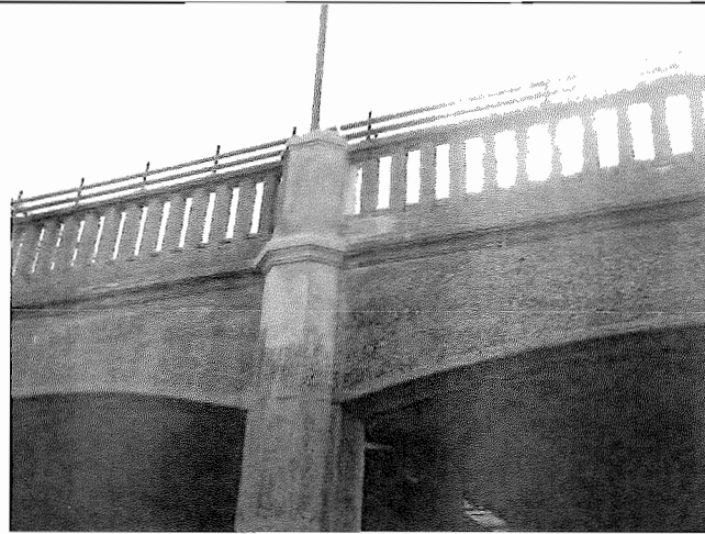
1. EAST ORANGE STATION BALUSTRADE REPAIRED
