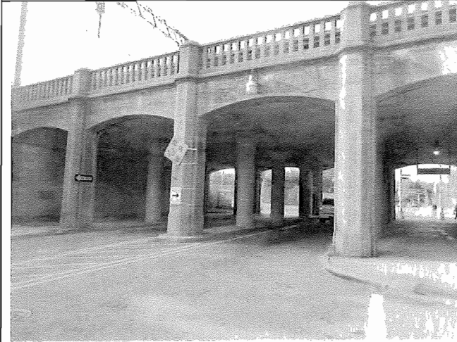
27. UNDERPASS AT SO MUNN AVE & CITY HALL PLAZA
