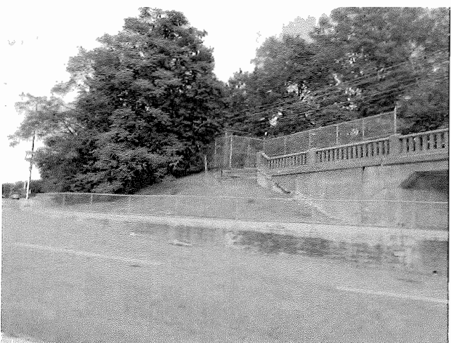
5. RETAINING WALL REPAIRED
