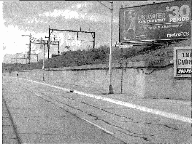
26. RETAINING WALL ALONG FREEWAY DRIVE EAST
