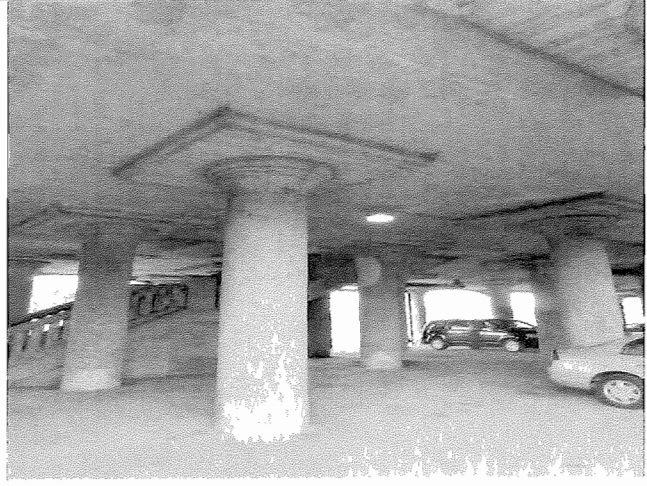
28. PILLARS UNDER EAST ORANGE TRAIN STATION
