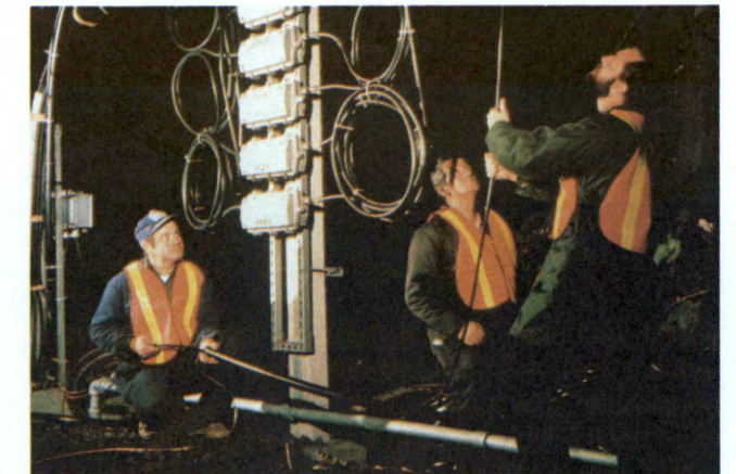
A link in the Teleport network: Installing fiber optic cable in a PATH tunnel.
