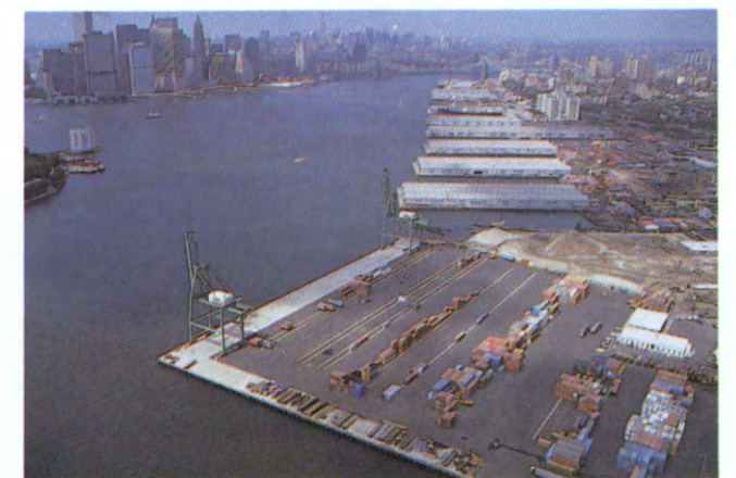
Modernizing the Brooklyn waterfront: The expanding Red Hook Container Terminal.
