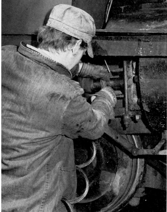
Bob Morris repacks bearings on "Lady Edith," a steam locomotive dating back to 1887. Lady Edith was imported from Ireland, where it ran until the 1950's on the Cavan and Leitram Railroad.
