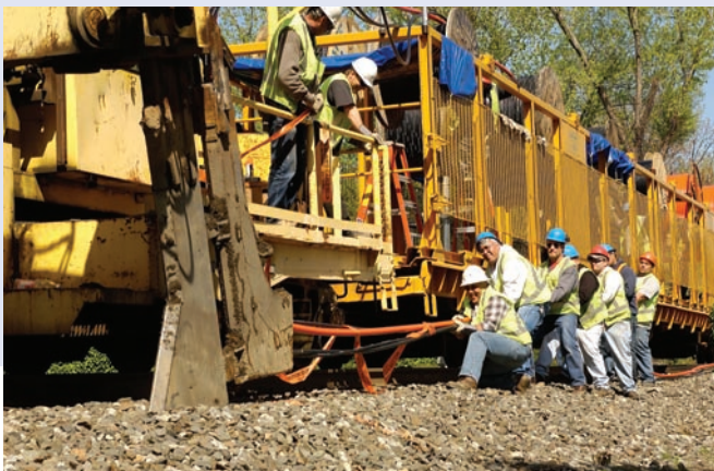
Workers install signal cable along the Pascack Valley Line.
